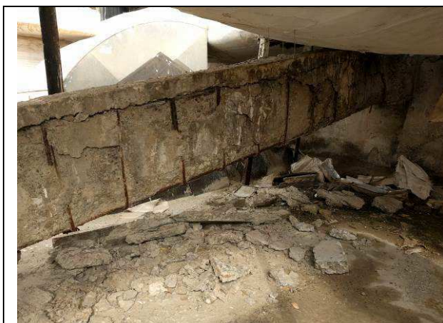
Fig. 1- Corrosion and deterioration of concrete beam
