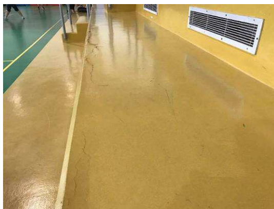
Fig. 14- Cracks on the seating area
