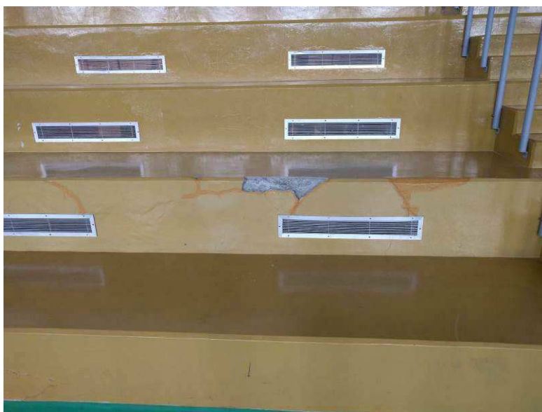
Fig. 17- New seating area cracks
