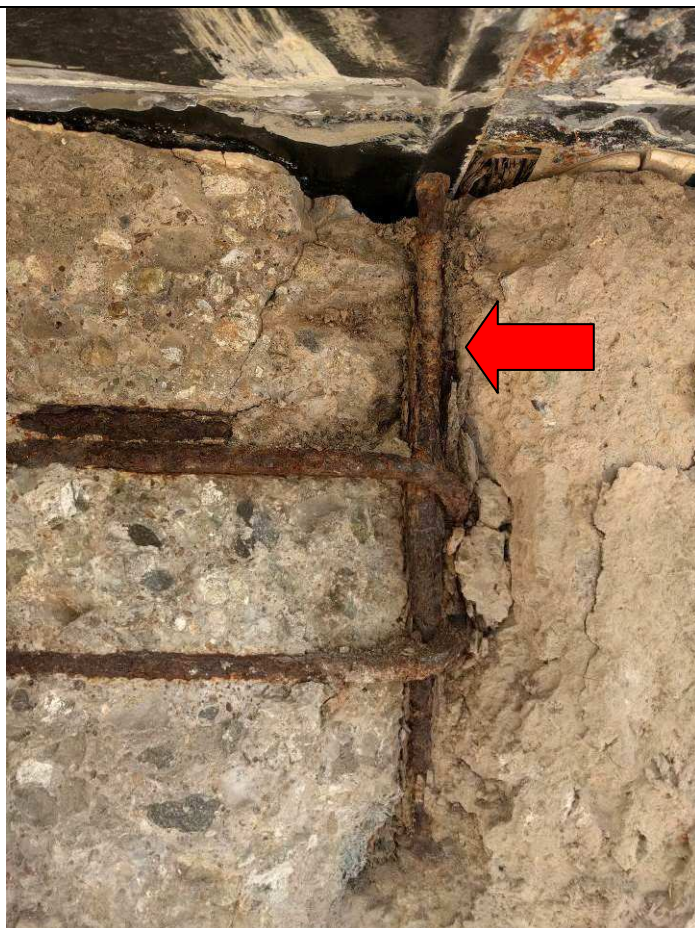
Fig. 13- Steel elements lost part of their section
