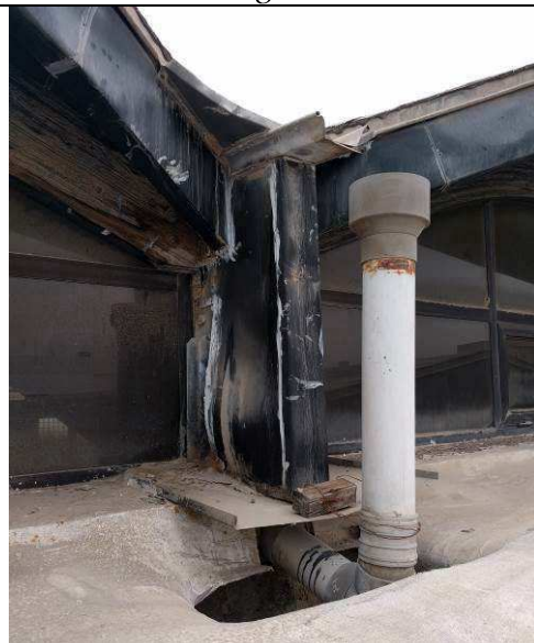
Fig. 10- Water evacuation and wood beam protection defect
