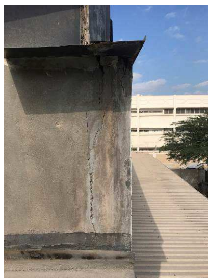
Fig. 11- Crack at the edge of the beam
