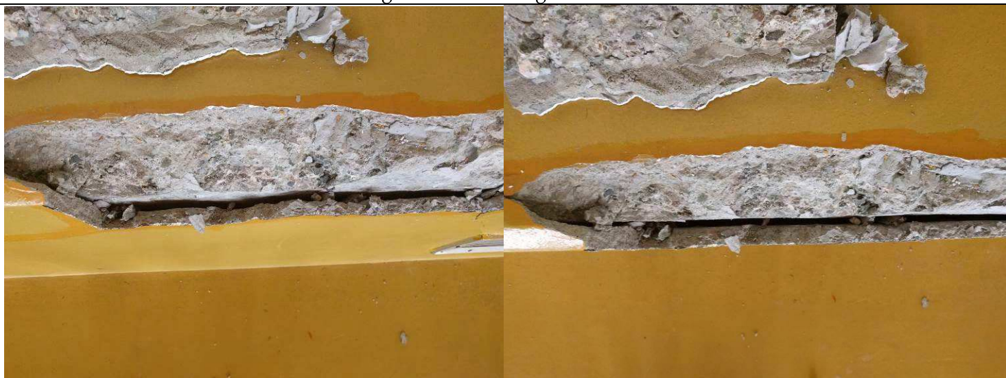
Fig. 17- New seating area cracks
