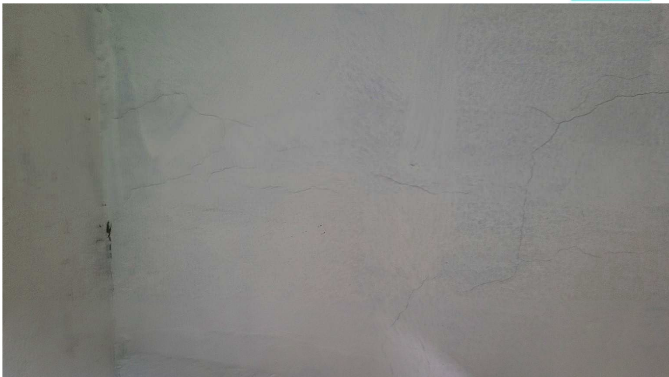
Figure 4-65 Crack in stands soffit
