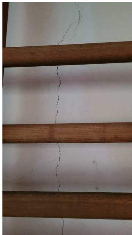
Figure 4-42 cracks in block wall
