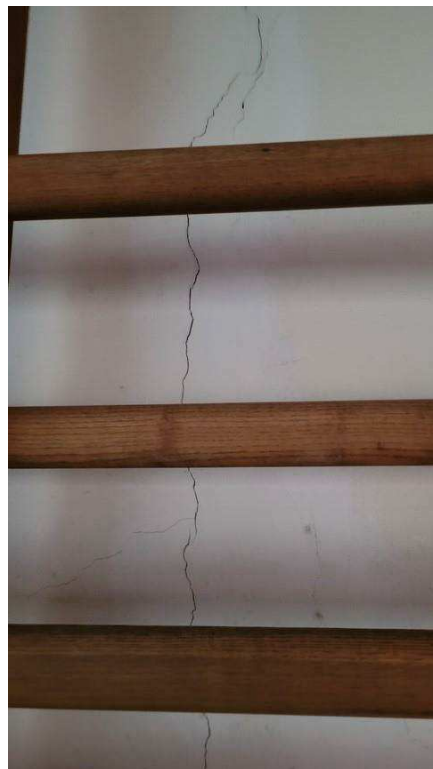
Figure 4-42 Cracks in block wall
