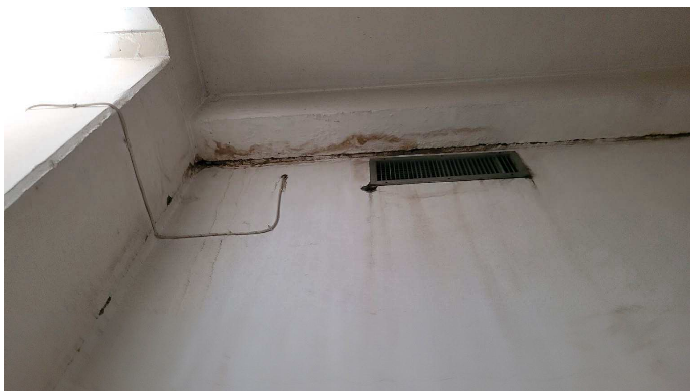
Figure 4-80 previous leakage at expansion joint
