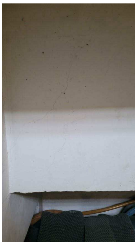
Figure 4-72 Cracks in stands soffit
