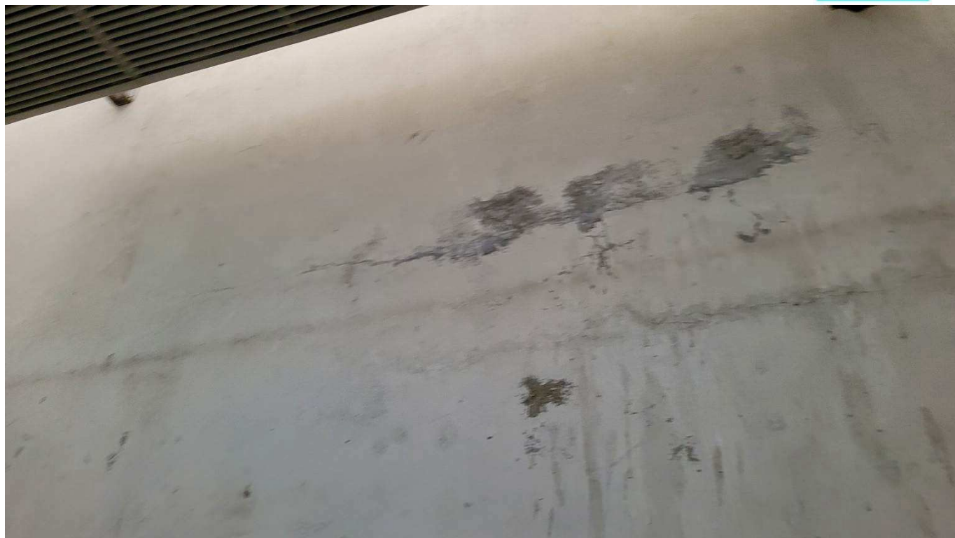
Figure 4-77 Cracks and dampness in wall
