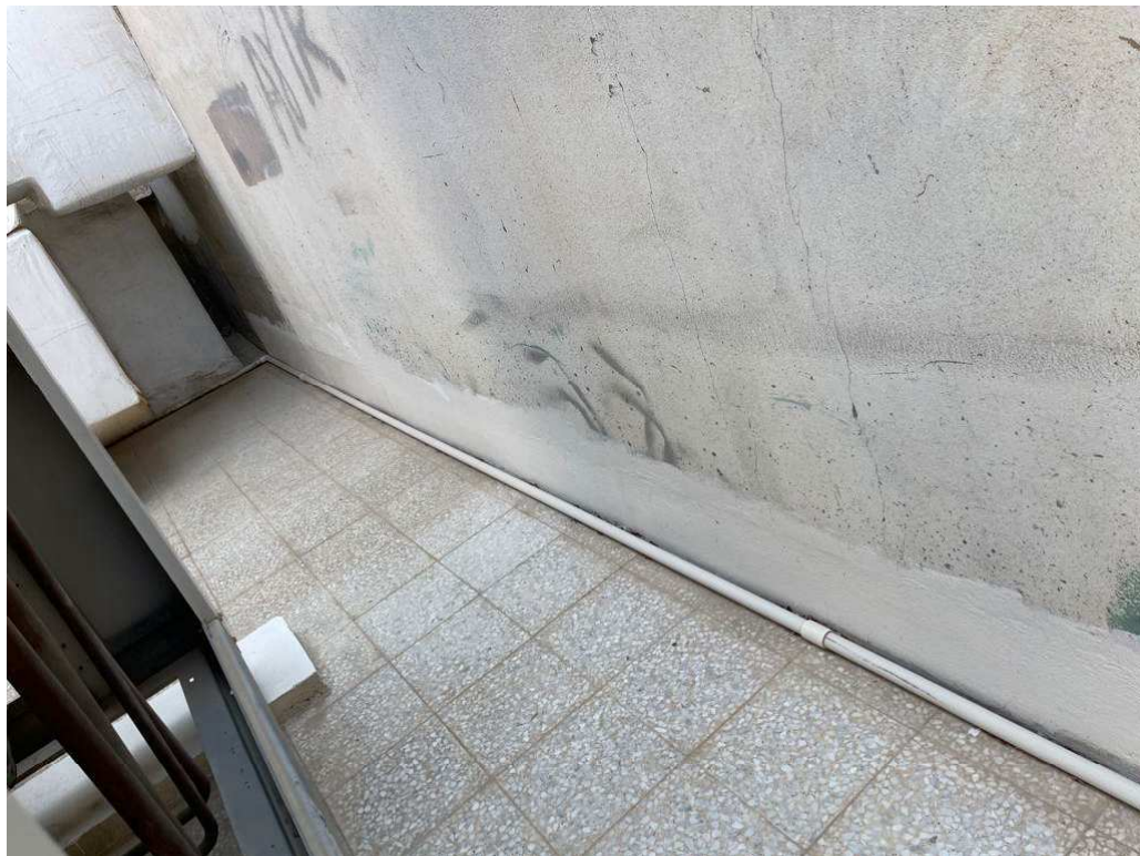
Figure 4-20 Cracks between block walls and concrete elements
