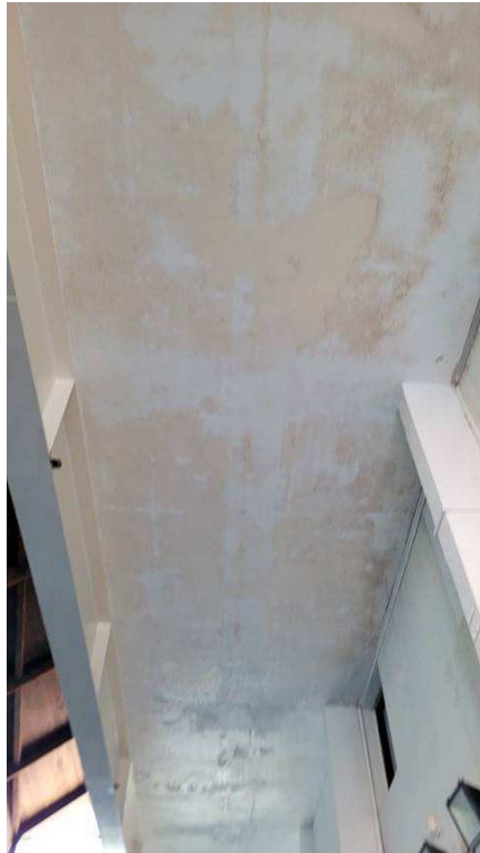
Figure 4-87 Previous leakage in slab soffit
