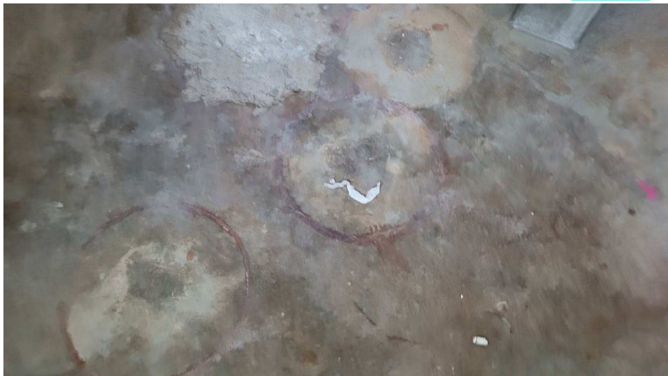
Figure 4-73 sign of previous leakage in flooring
