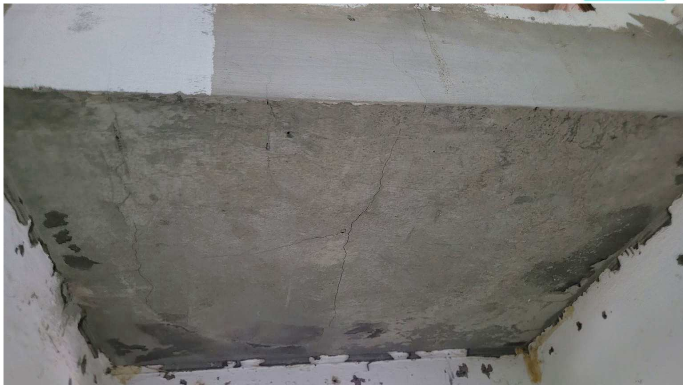
Figure 4-55 Delamination in stands soffit
