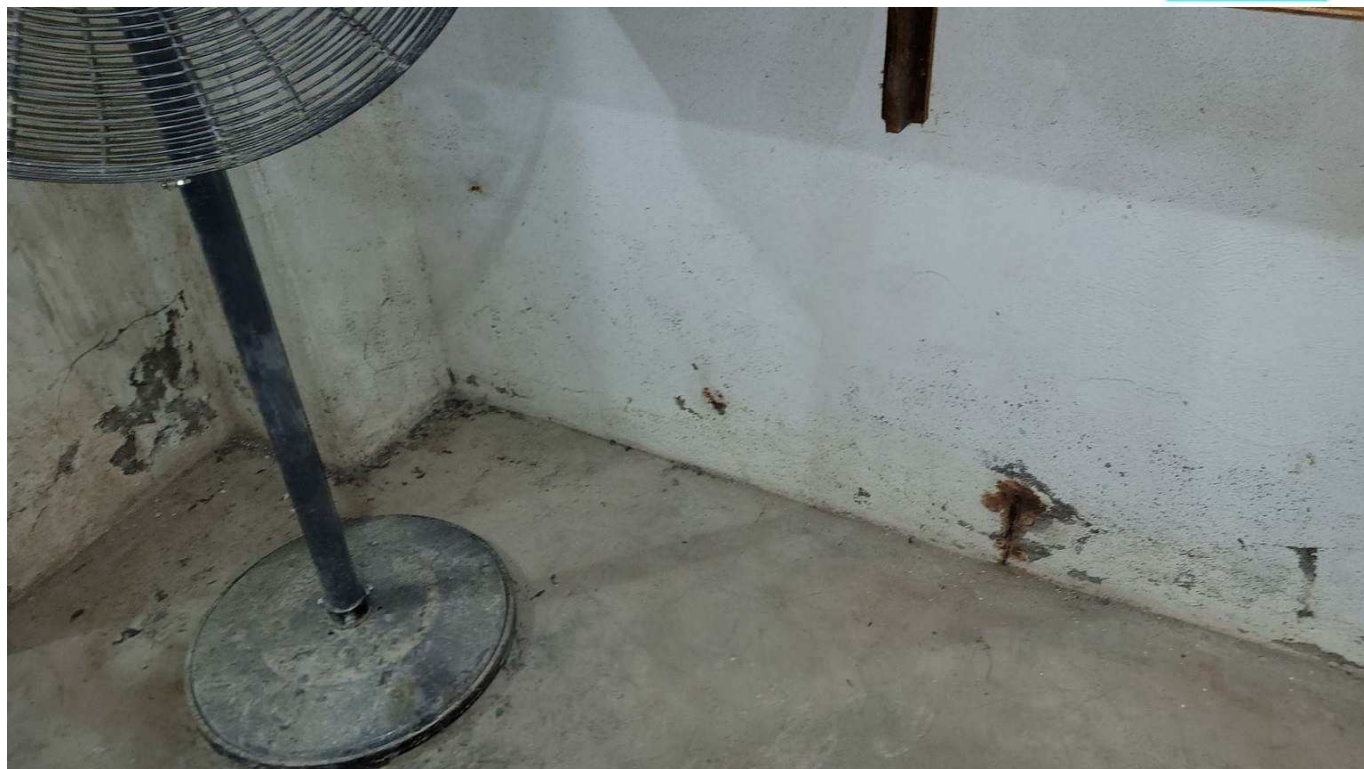
Figure 4-59 Delamination and previous leakage in concrete wall
