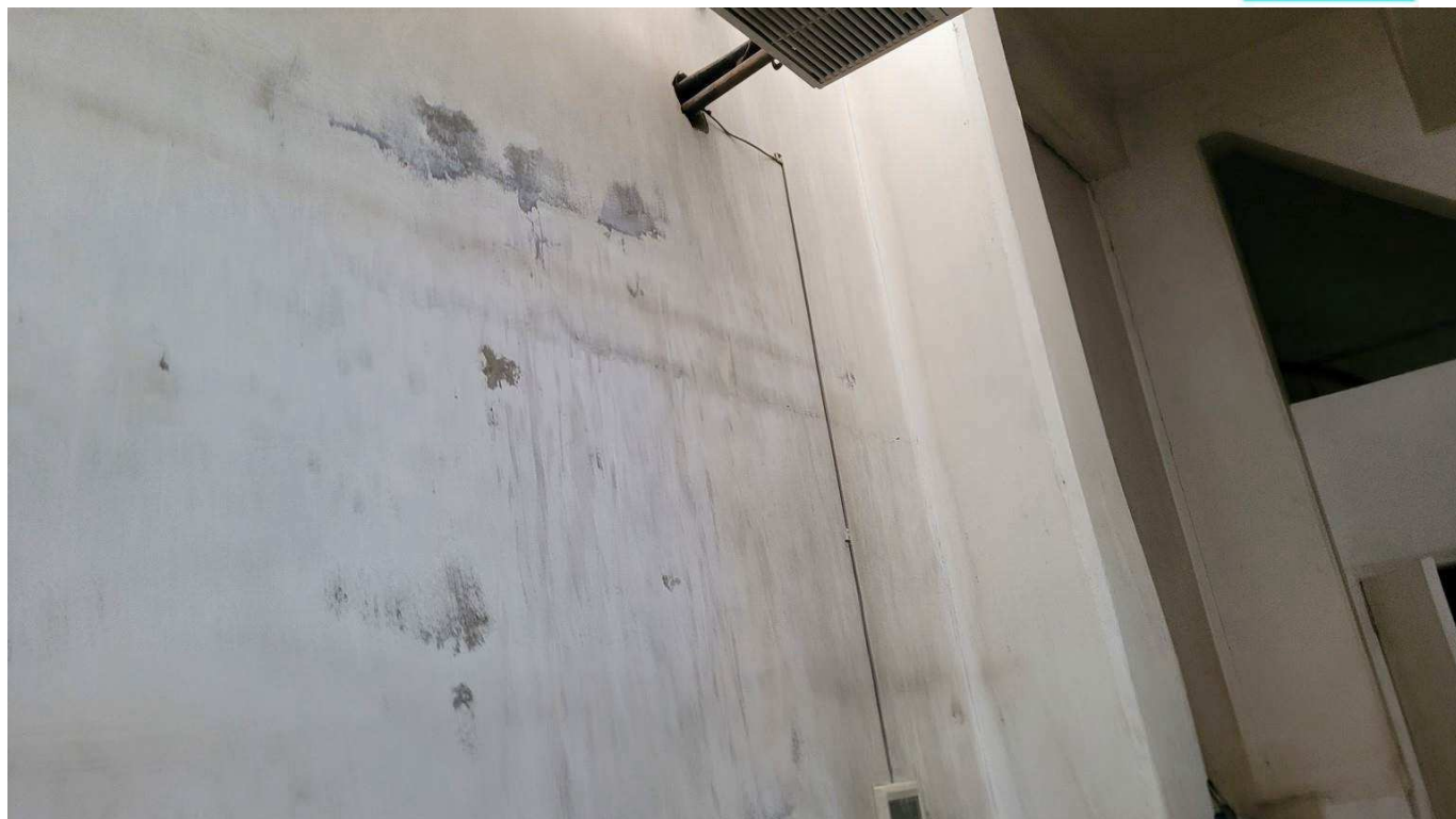
Figure 4-81 dampness and cracks in block wall
