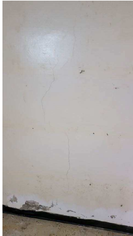
Figure 4-39 Dampness and cracks in block walls
