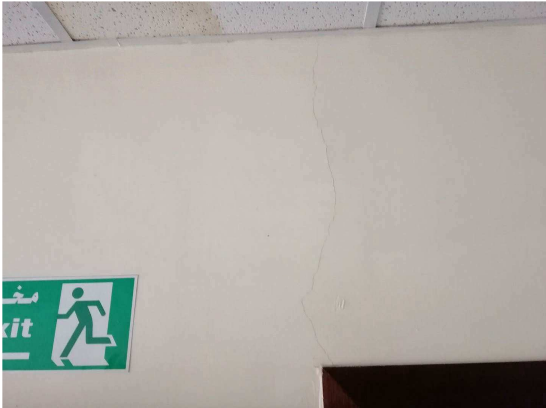
Figure 4-18 crack in block wall
