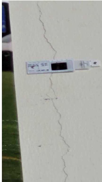
Figure 4-49 Crack in concrete wall
