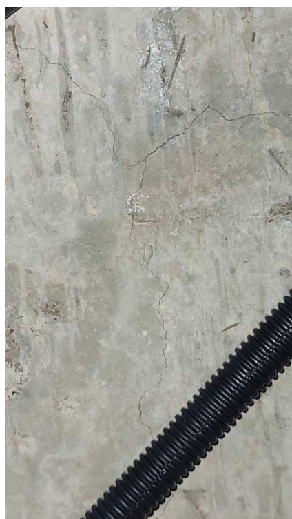
Figure 4-8 Cracks in slab soffit
