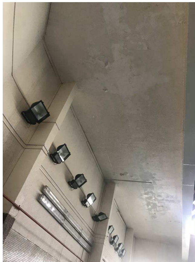
Figure 4-43 Dampness in slab soffit
