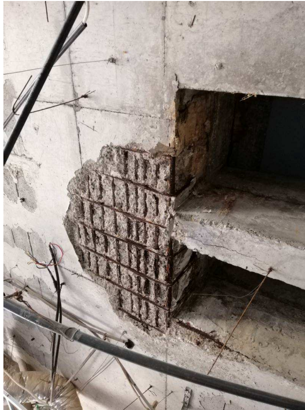
Figure 4-2 spalled cover and corroded steel at the playing area slab soffit
