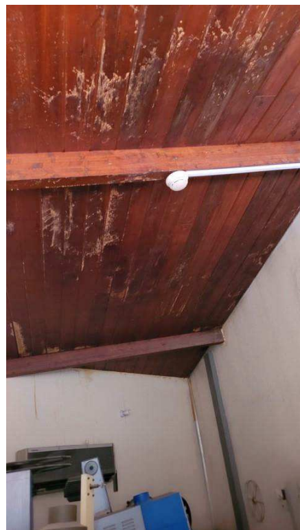
Figure 4-34 Previous leakage in wooden roof
