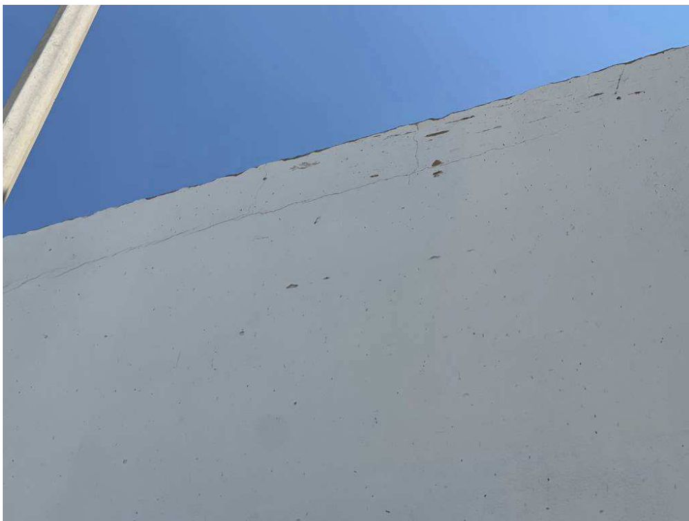
Figure 4-24 Crack between block wall and slab
