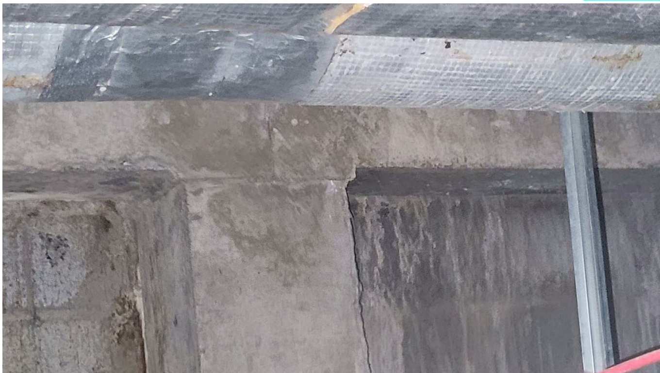
Figure 4-13 Previous leakage in beam and block wall
