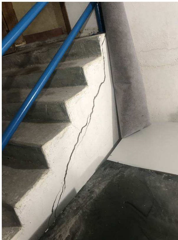
Figure 4-35 crack in staircase
