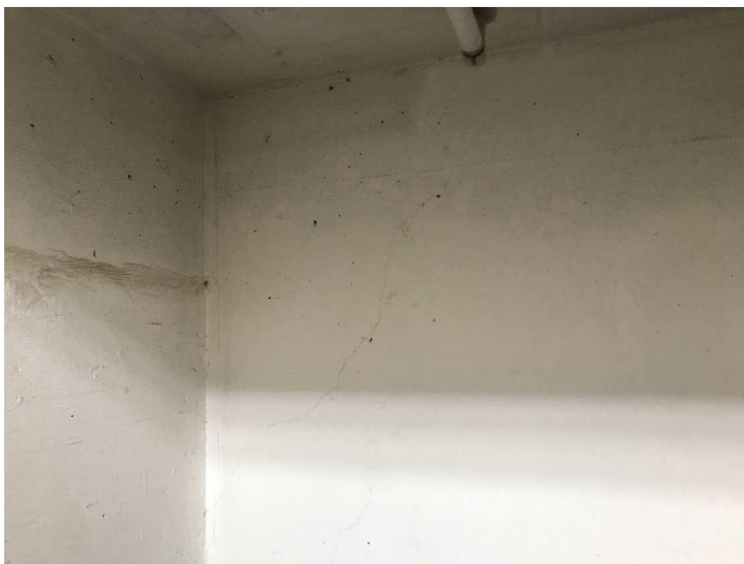
Figure 4-37 Cracks in concrete wall
