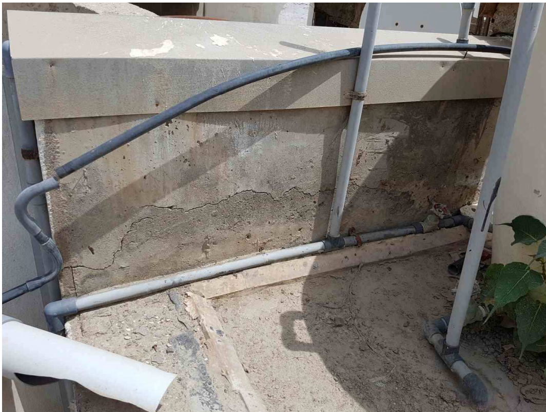
Figure 4-7 Cracks in beam due to steel reinforcement corrosion
