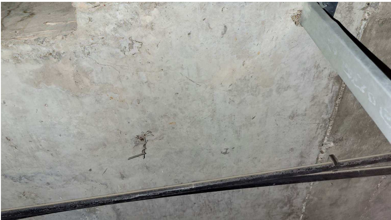
Figure 4-32 cracks in slab soffit
