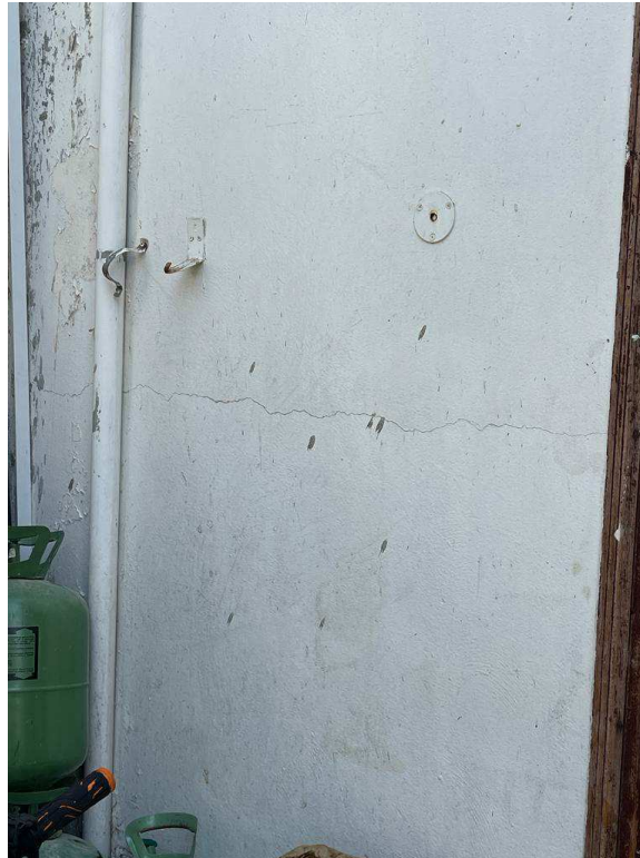
Figure 4-25 Crack in block walls
