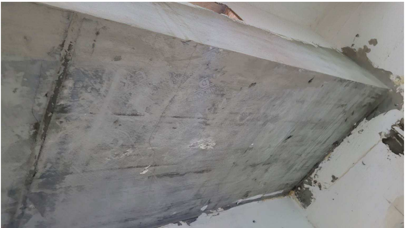
Figure 4-56 Cracks in stands soffit
