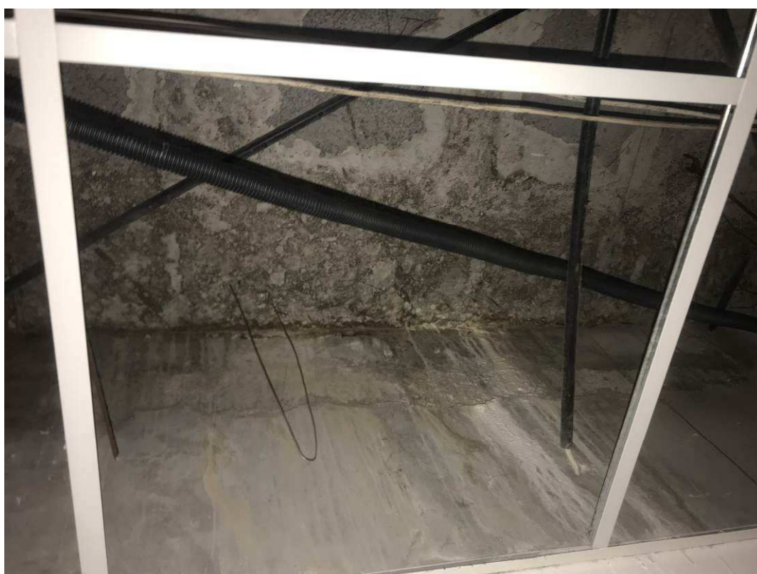
Figure 4-11 sign of previous leakage
