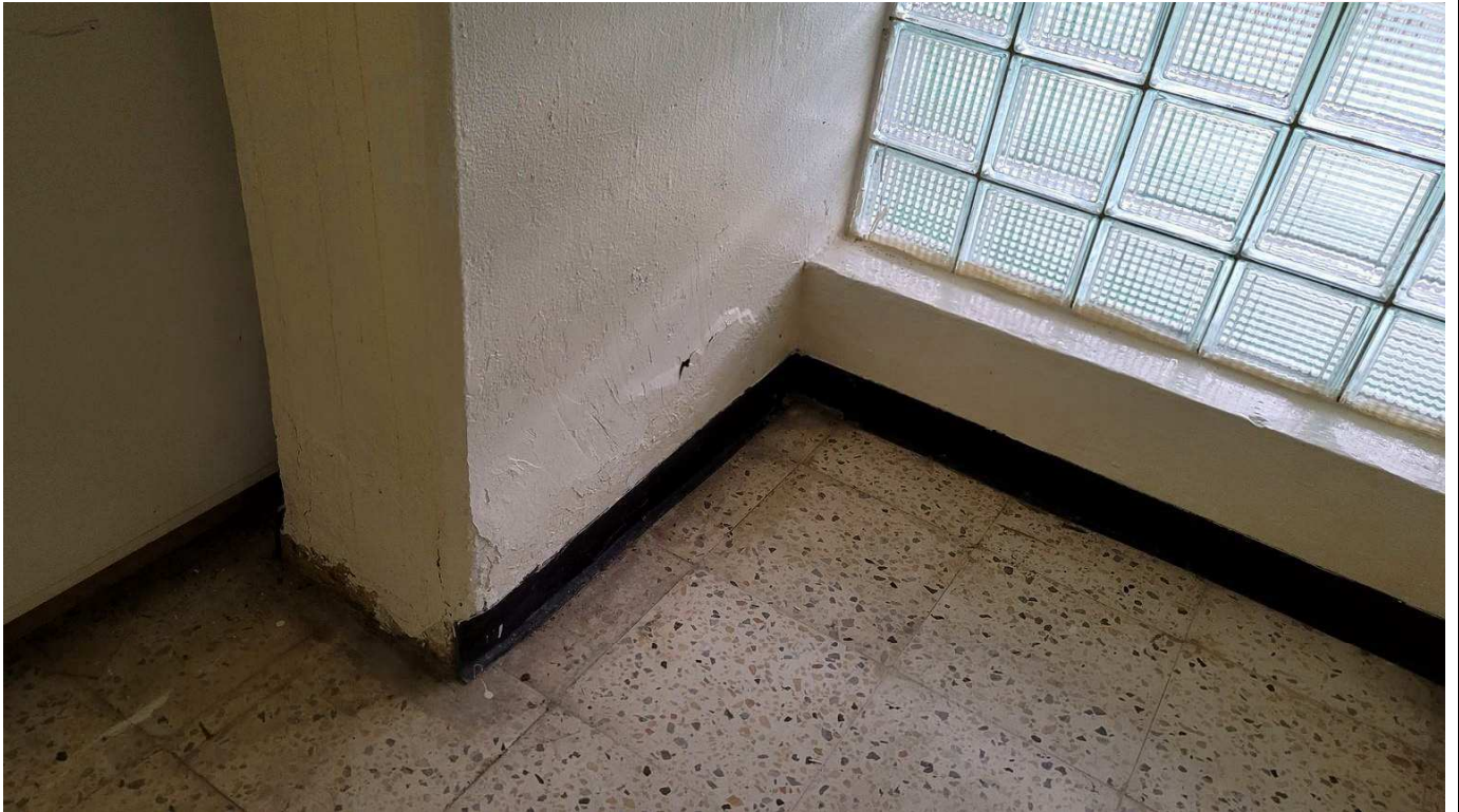
Figure 4-37 delamination in column
