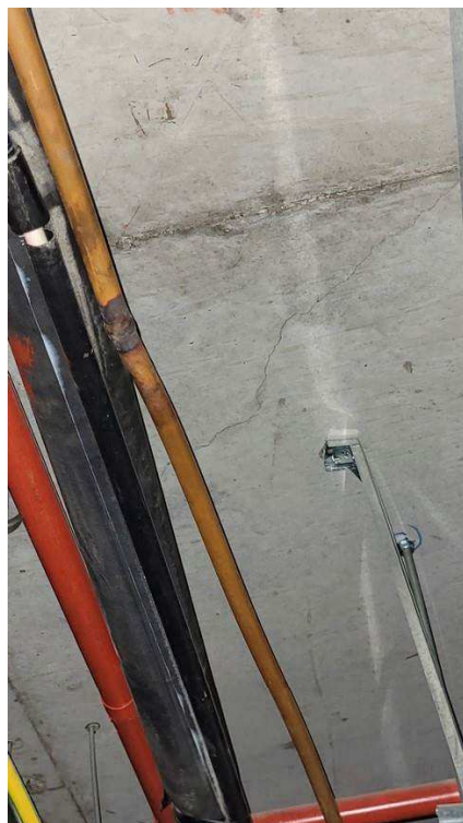
Figure 4-7 Cracks in slab soffit
