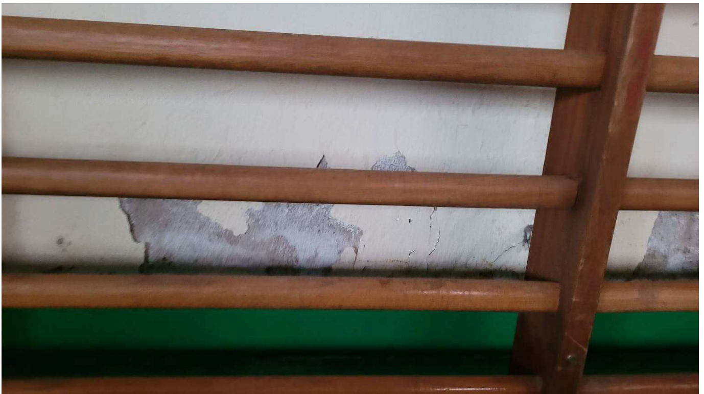
Figure 4-44 Dampness and delamination in ground beam
