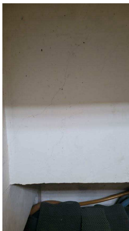
Figure 4-72 Cracks in stands soffit
