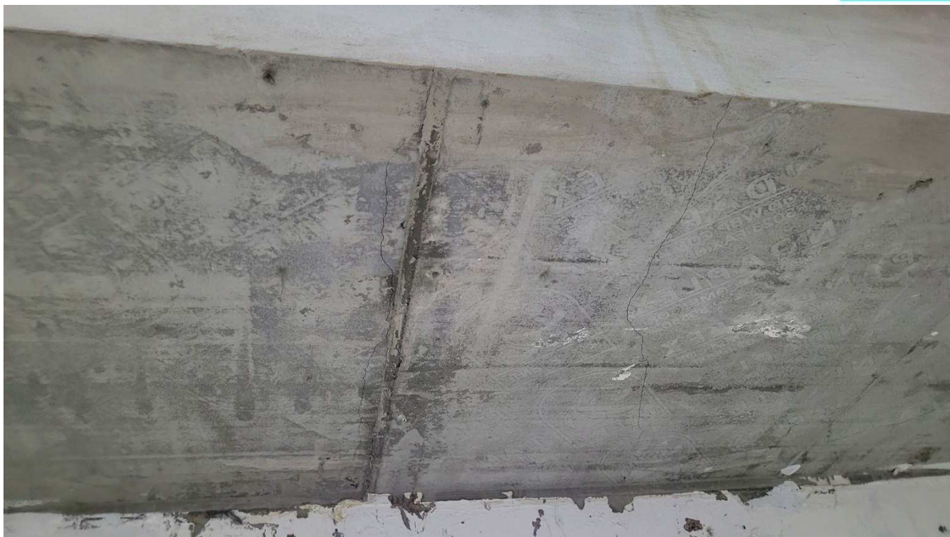
Figure 4-53 Cracks in stands soffit
