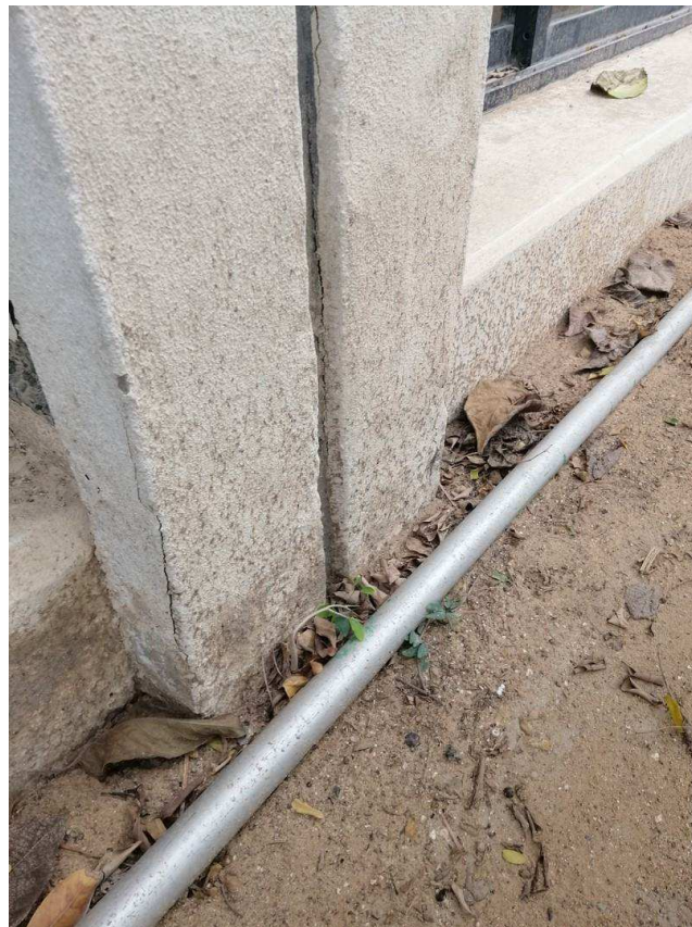
Figure 4-15 Cracks in column due to steel corrosion
