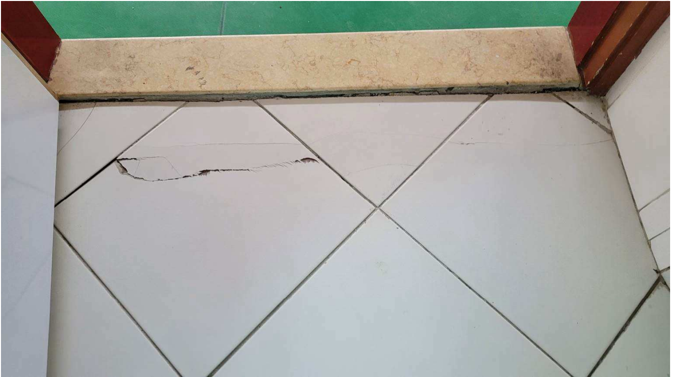
Figure 4-47 Cracks in tiles in toilets in the gym
