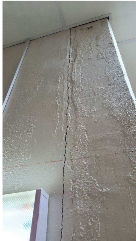
Figure 4-41 Crack between block wall and concrete element
