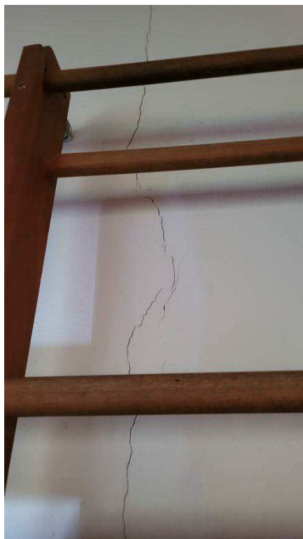
Figure 4-43 Cracks in block wall
