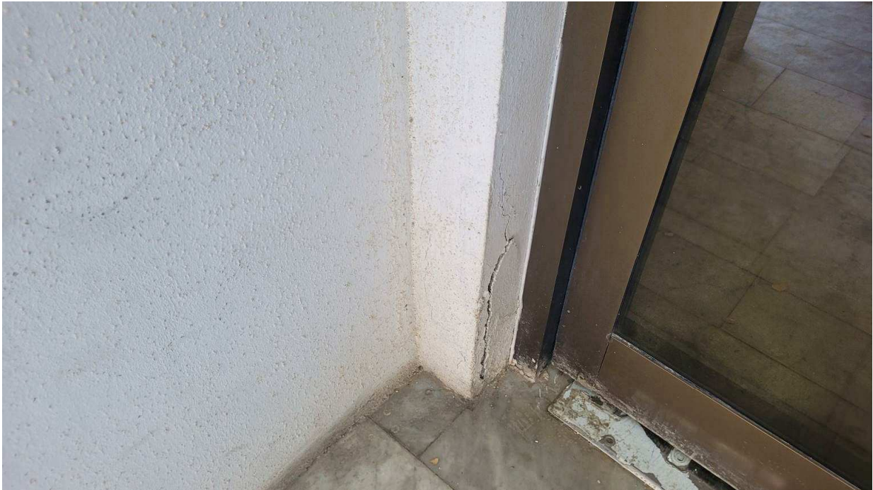
- Figure 4-1 Delamination in column
