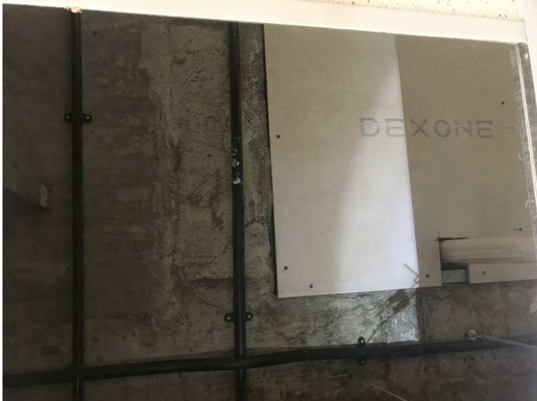
Figure 4-23 slab opening which not closed properly
