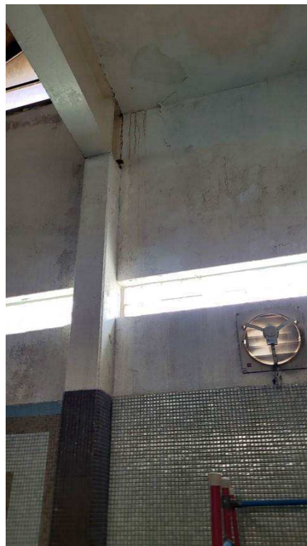
Figure 4-84 Dampness in block wall and concrete elements
