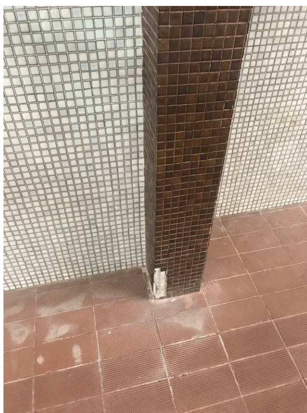
Figure 4-39 delamination in column
