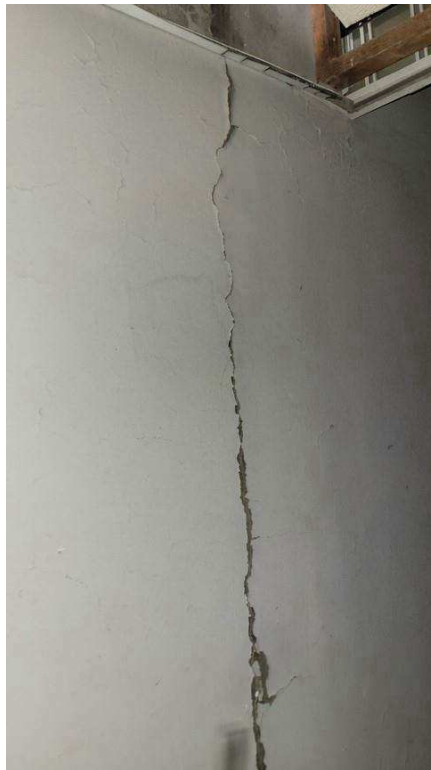
Figure 4-12 Crack between block wall and concrete element
