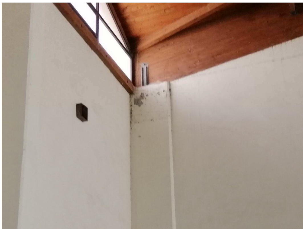
Figure 4-53 delamination and corrosion in column
