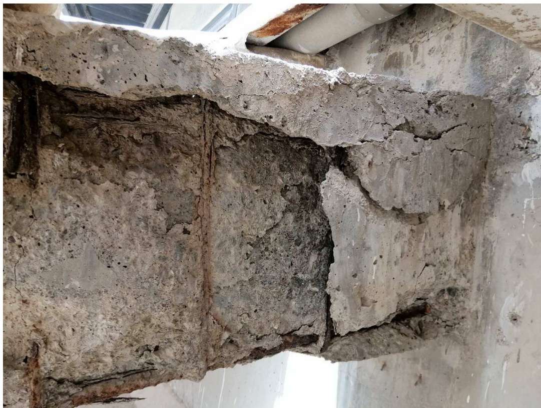
Figure 4-4 spalled cover and corroded steel at the playing area roof
