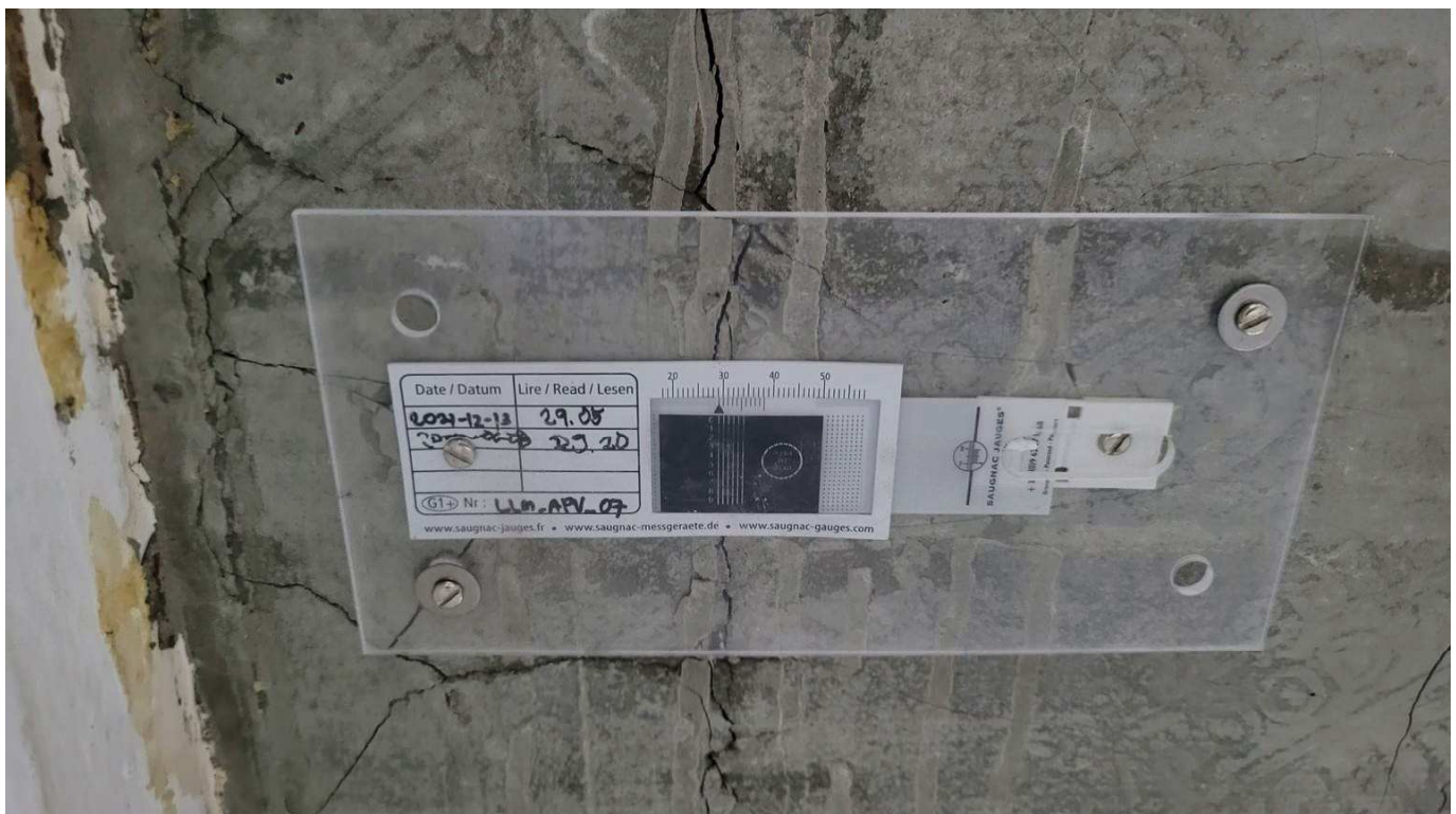
Figure 4-52 Cracks and delamination of the concrete cover in concrete wall below stands
