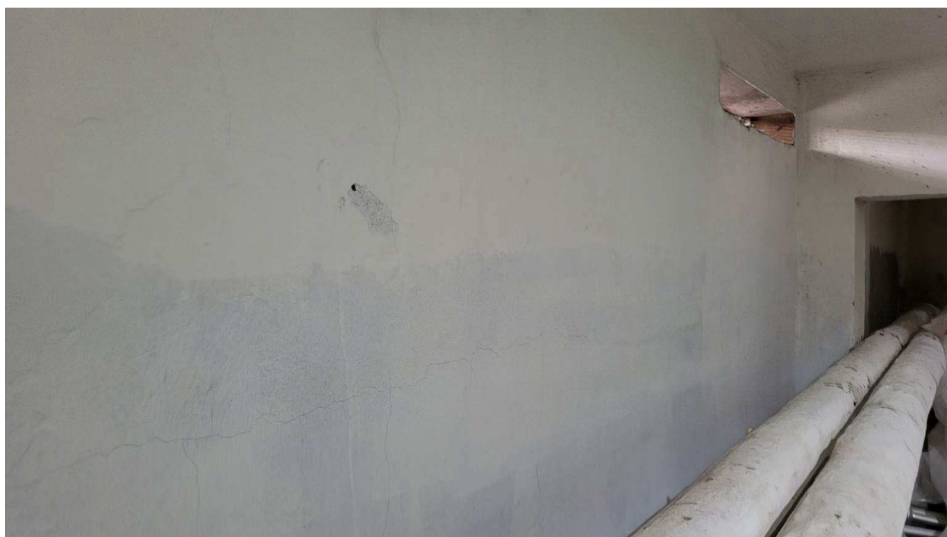
Figure 4-64 Crack in concrete wall
