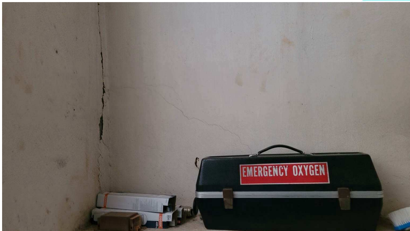
Figure 4-79 Crack in block wall
