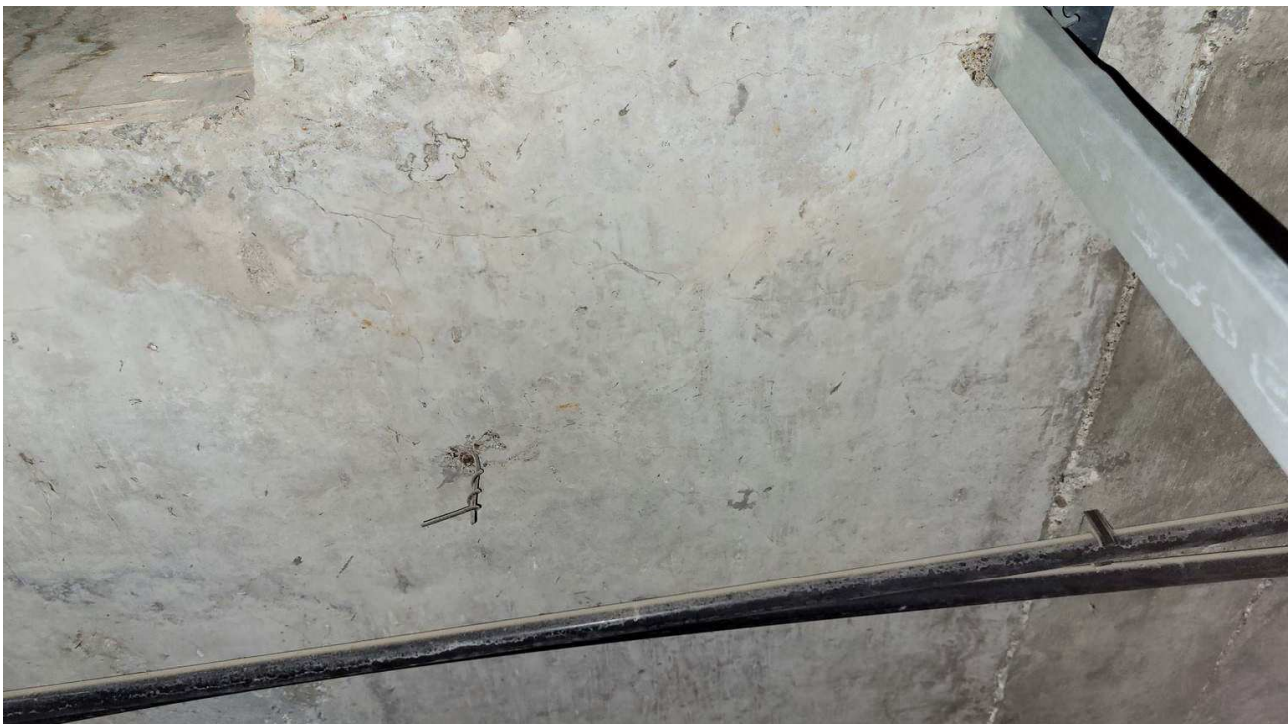
Figure 4-32 cracks in slab soffit
