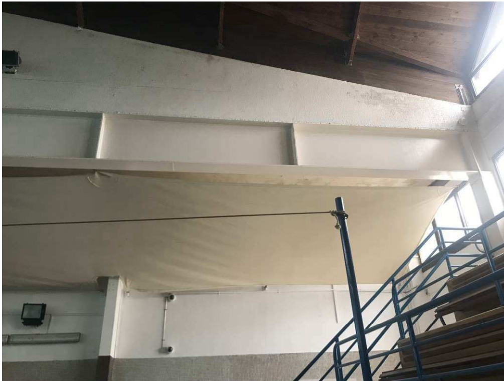
Figure 4-42 Dampness in slab soffit
