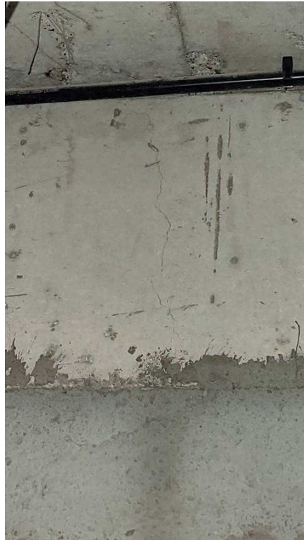
Figure 4-15 Crack in beam
