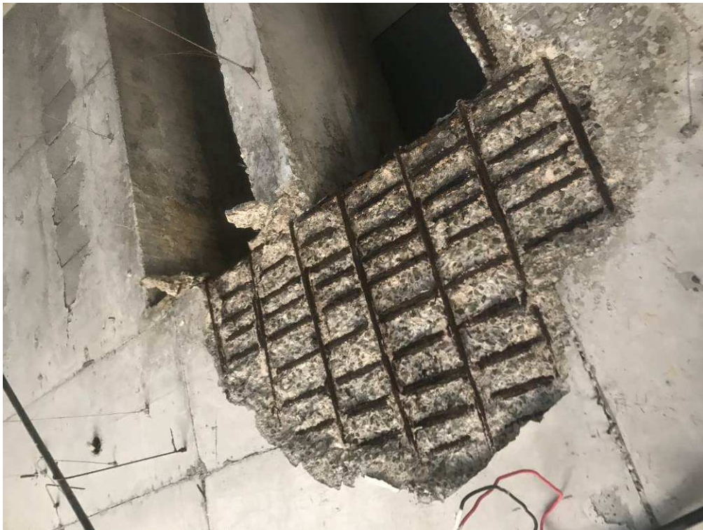
Figure 4-1 spalled cover and corroded steel at the playing area slab soffit
