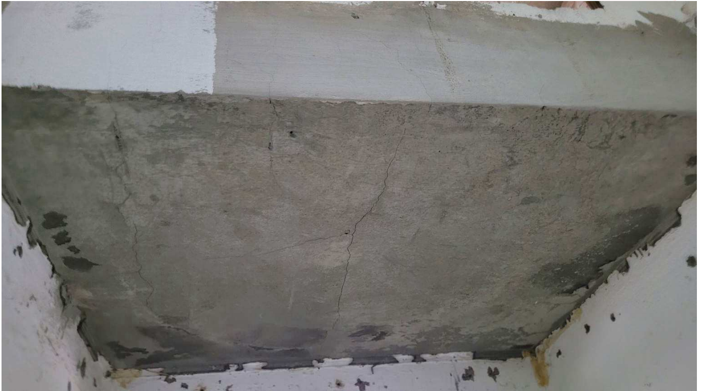
Figure 4-55 Delamination of the concrete cover in the stand's soffit
