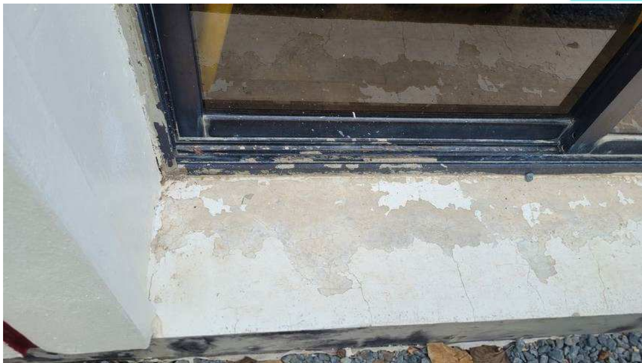
- Figure 4-3 Dampness and cracks in ground beam
