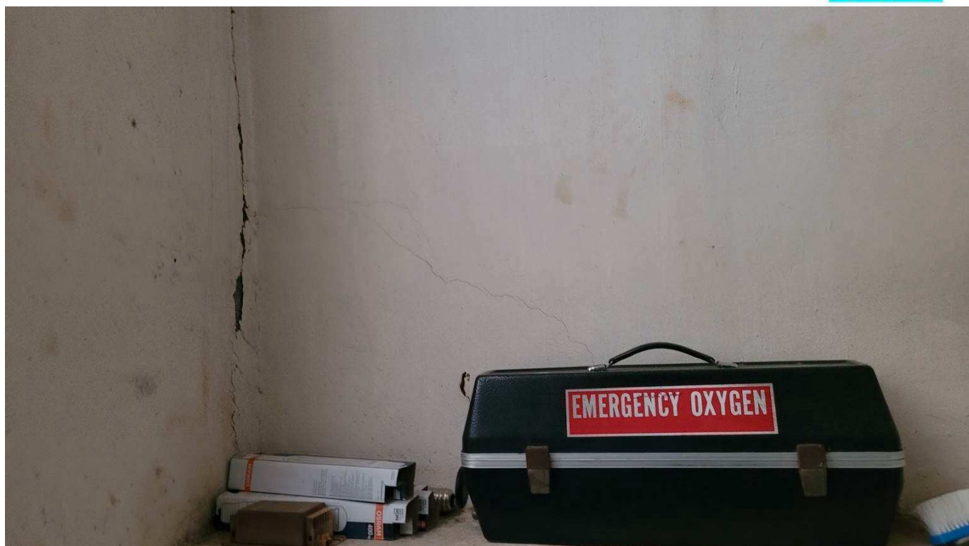
Figure 4-79 Crack in block wall
