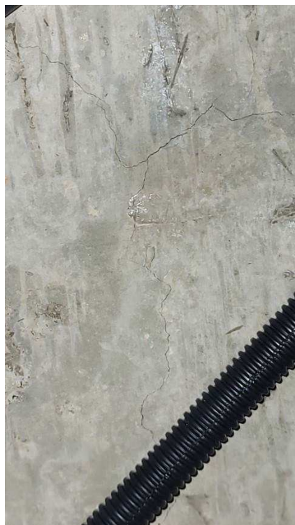
Figure 4-8 Cracks in slab soffit
