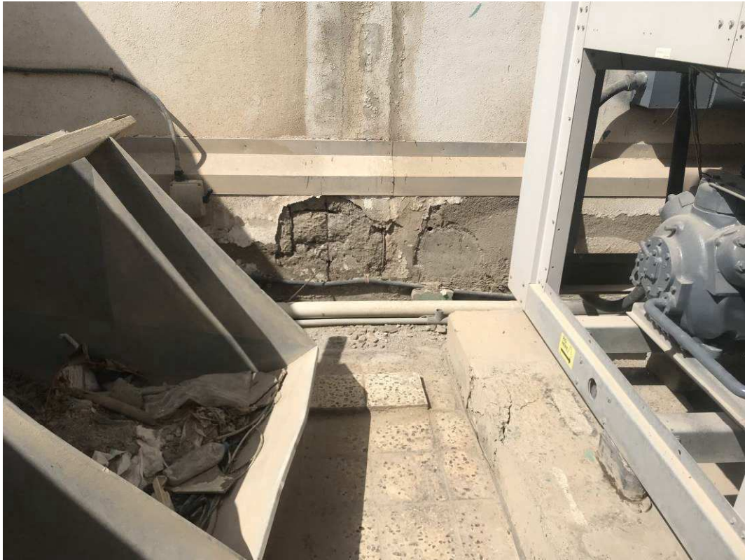
Figure 4-49 delamination and corrosion
