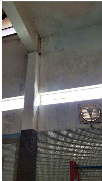
Figure 4-84 dampness in block wall and concrete elements
