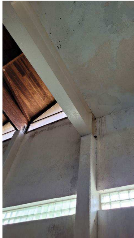
Figure 4-83 dampness in block walls and concrete elements
