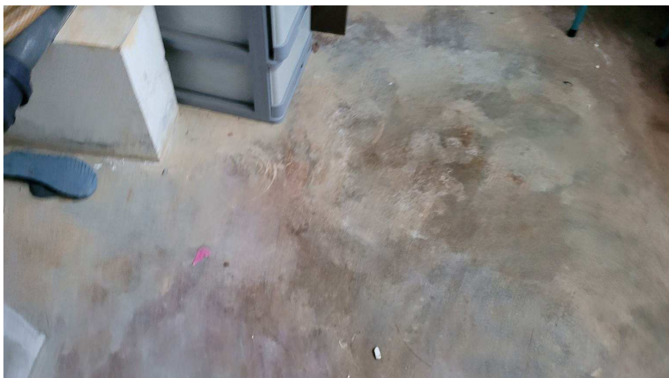
Figure 4-74 Sign of previous leakage in flooring
