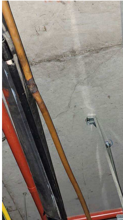
Figure 4-7 Cracks in slab soffit
