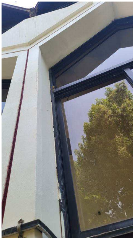
- Figure 4-2 Delamination in column
