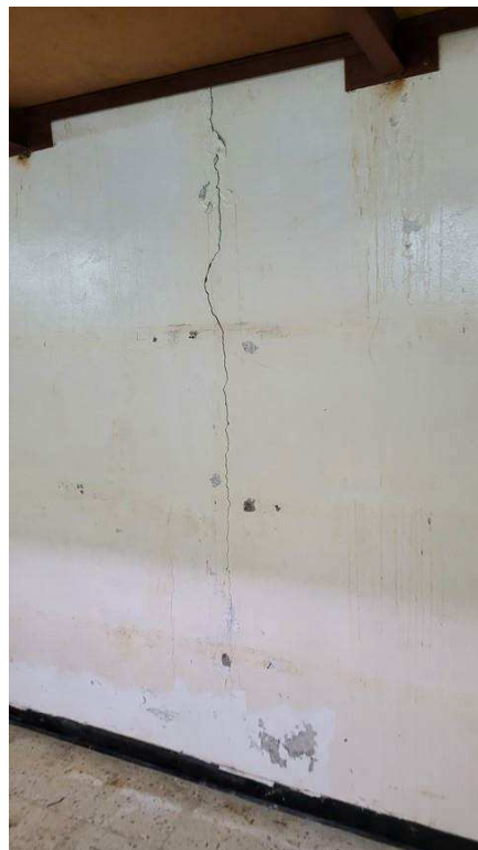
Figure 4-40 Dampness and cracks in block walls
