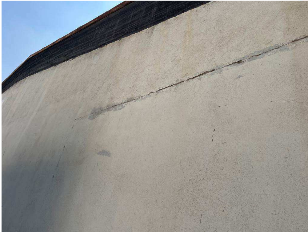
Figure 4-23 Crack between block wall and concrete element
