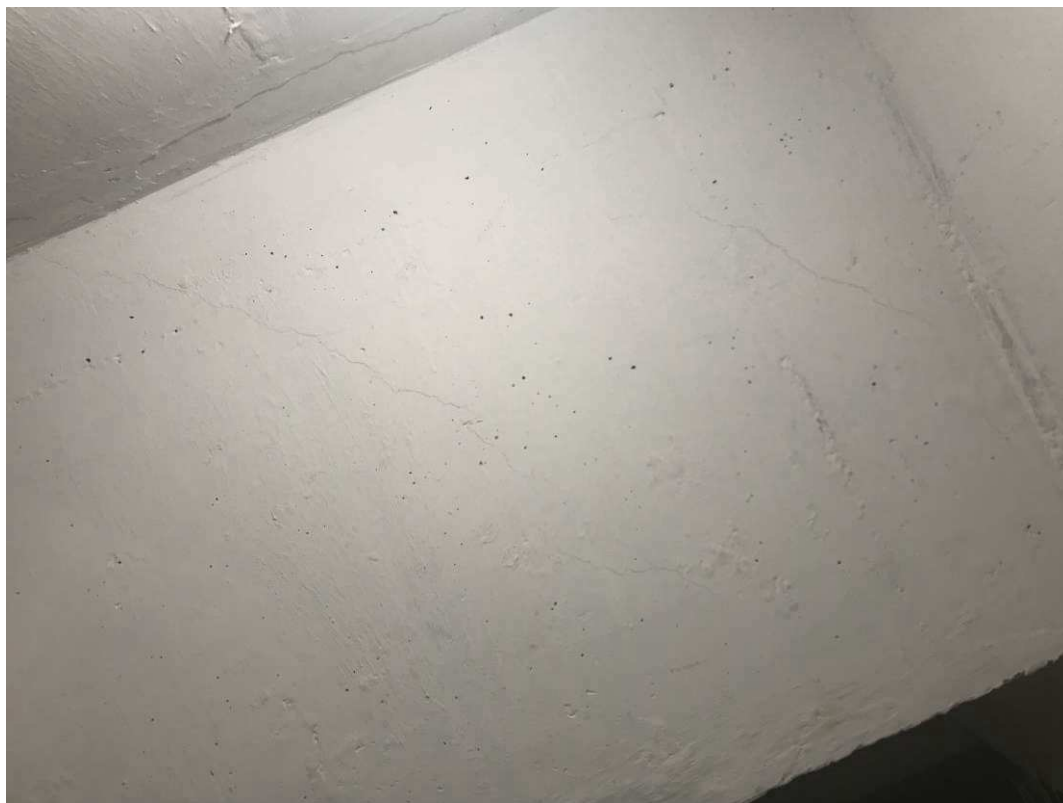
Figure 4-36 Cracks in concrete wall
