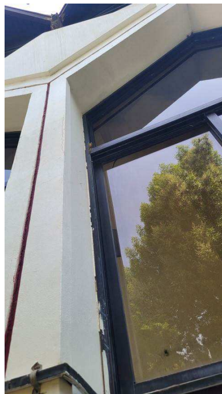
Figure 4-2 Delamination of the concrete cover in column
