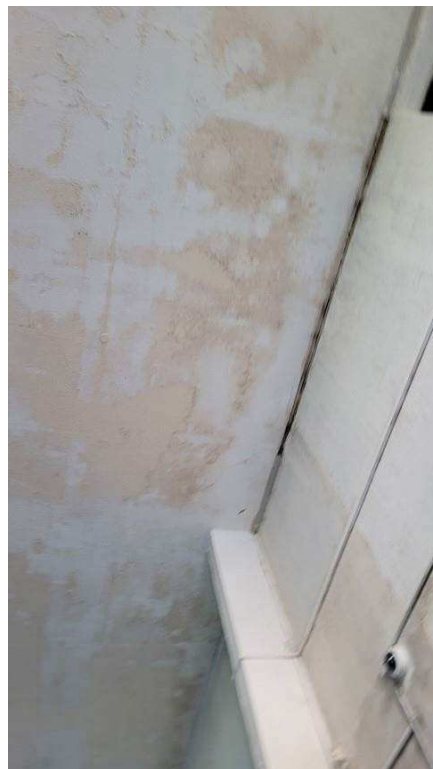
Figure 4-88 Previous leakage in slab soffit
