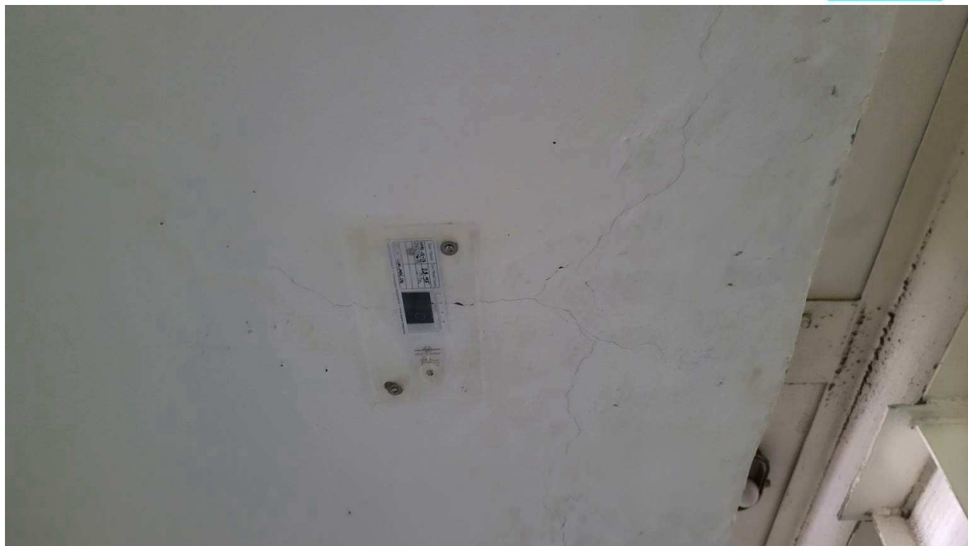
Figure 4-61 cracks in stands soffit
