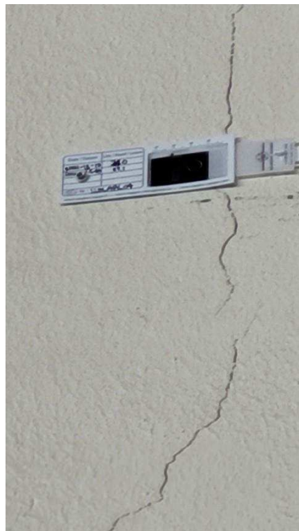
Figure 4-48 Crack in concrete wall
