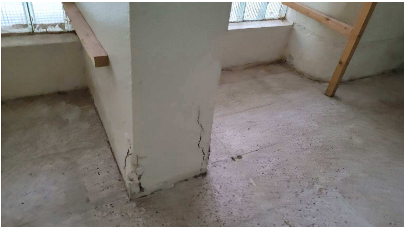
Figure 4-38 Delamination of the concrete cover in column
