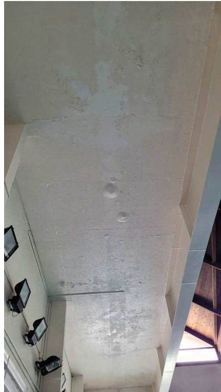
Figure 4-67 sign of previous leakage in slab soffit
