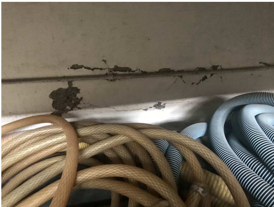
Figure 4-38 delamination in concrete wall
