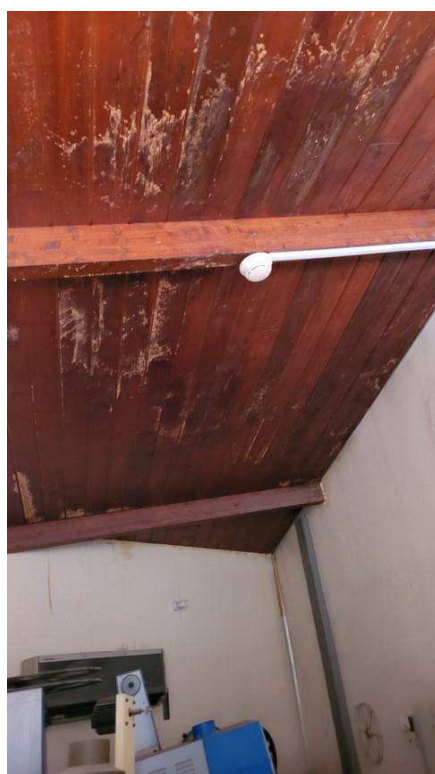
Figure 4-34 previous leakage in wooden roof
