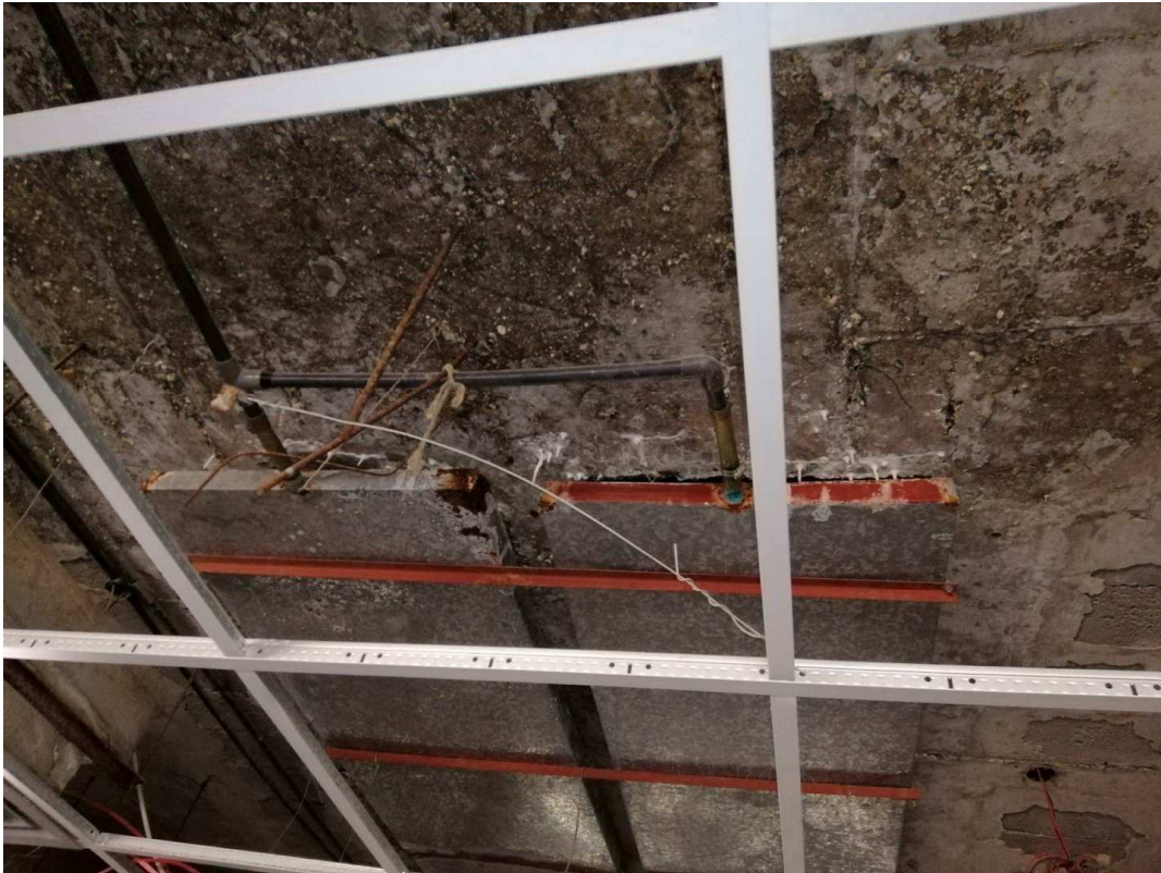
Figure 4-8 Delamination and sign of previous leakage
