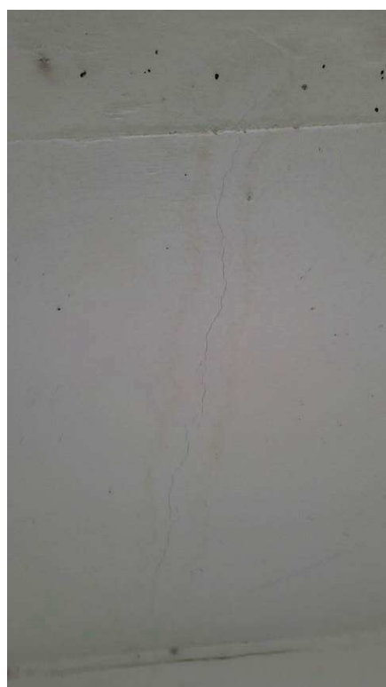
Figure 4-62 crack with previous leakage in stands soffit
