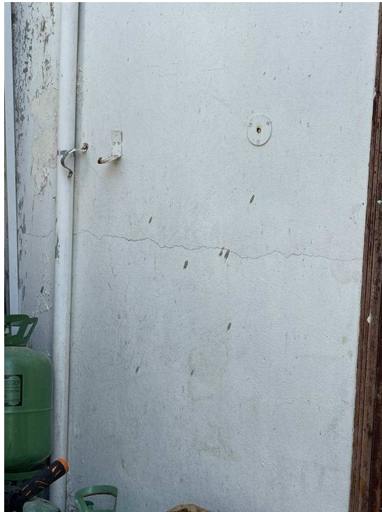
Figure 4-25 Crack between block wall
