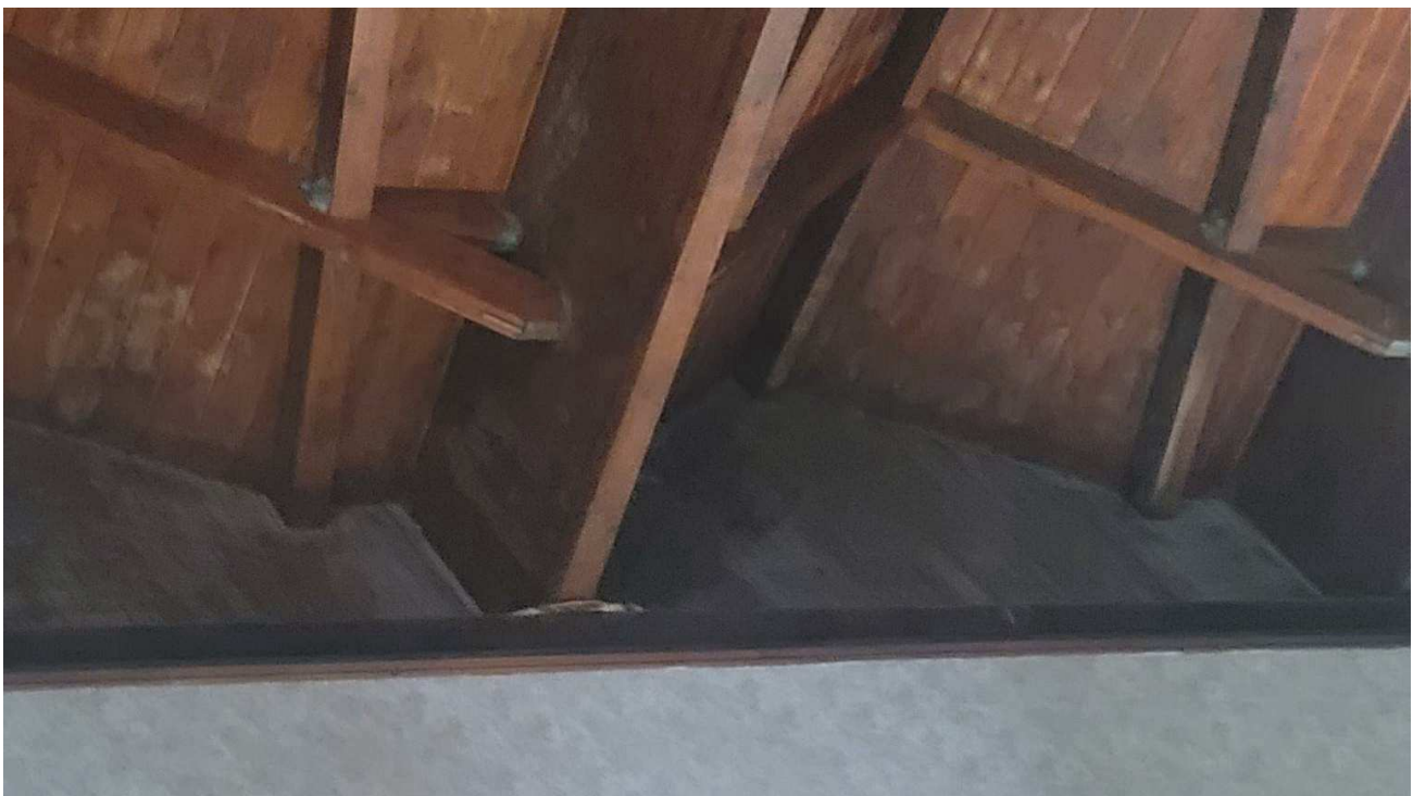
Figure 4-90 Previous leakage in slab soffit
