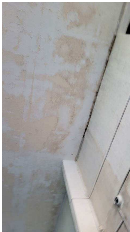
Figure 4-88 previous leakage in slab soffit
