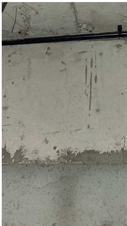
Figure 4-15 Crack in beam
