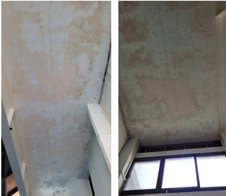
Figure 4-89 previous leakage in slab soffit
