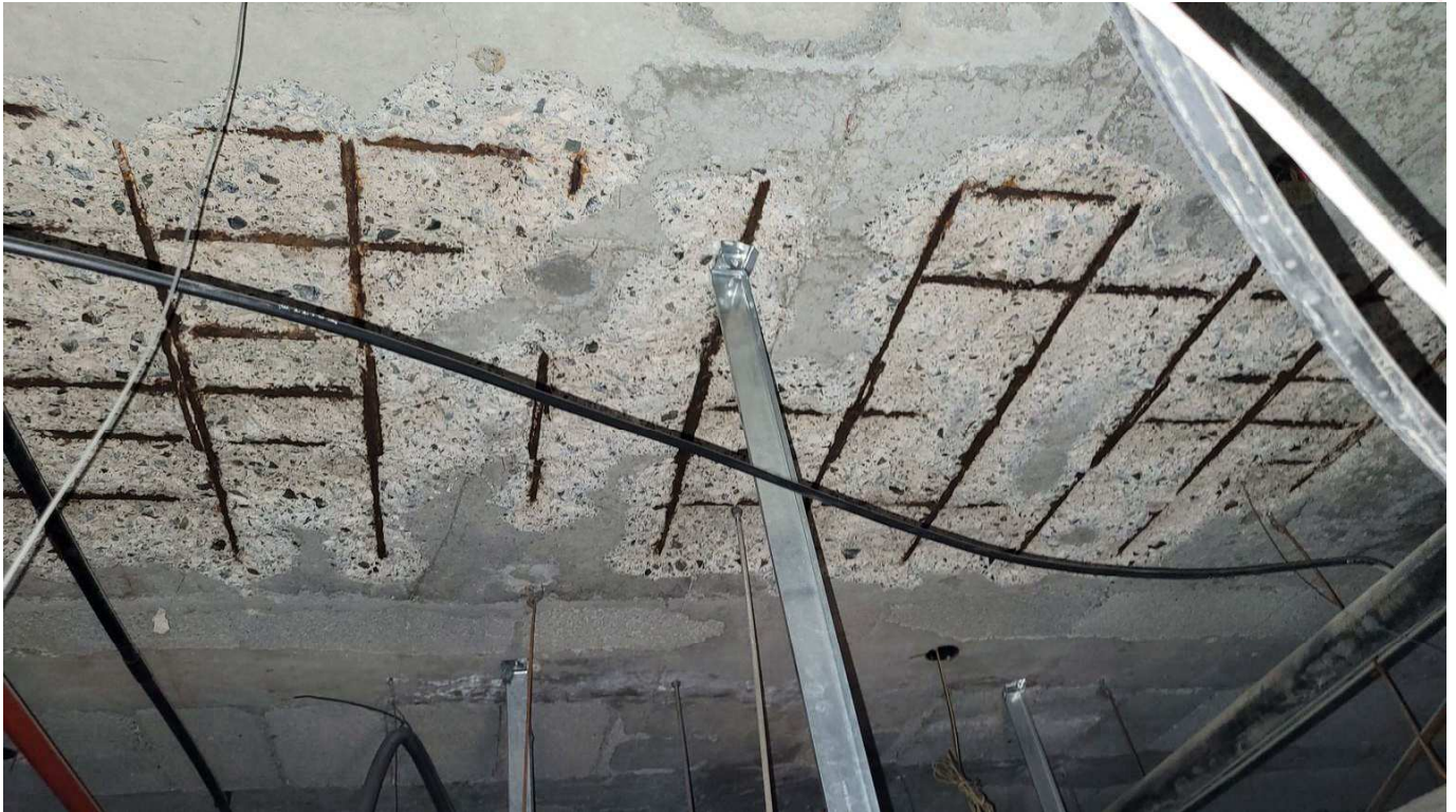
Figure 4-11 Steel exposure with corrosion in slab soffit
