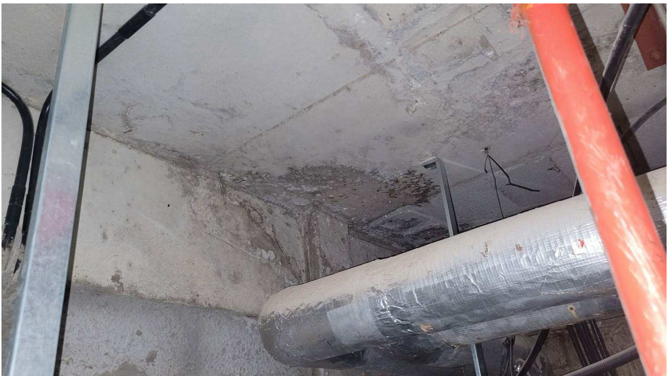
Figure 4-16 Previous leakage in beam and slab
