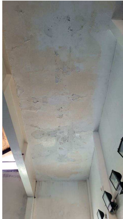
Figure 4-85 Previous leakage in slab soffit
