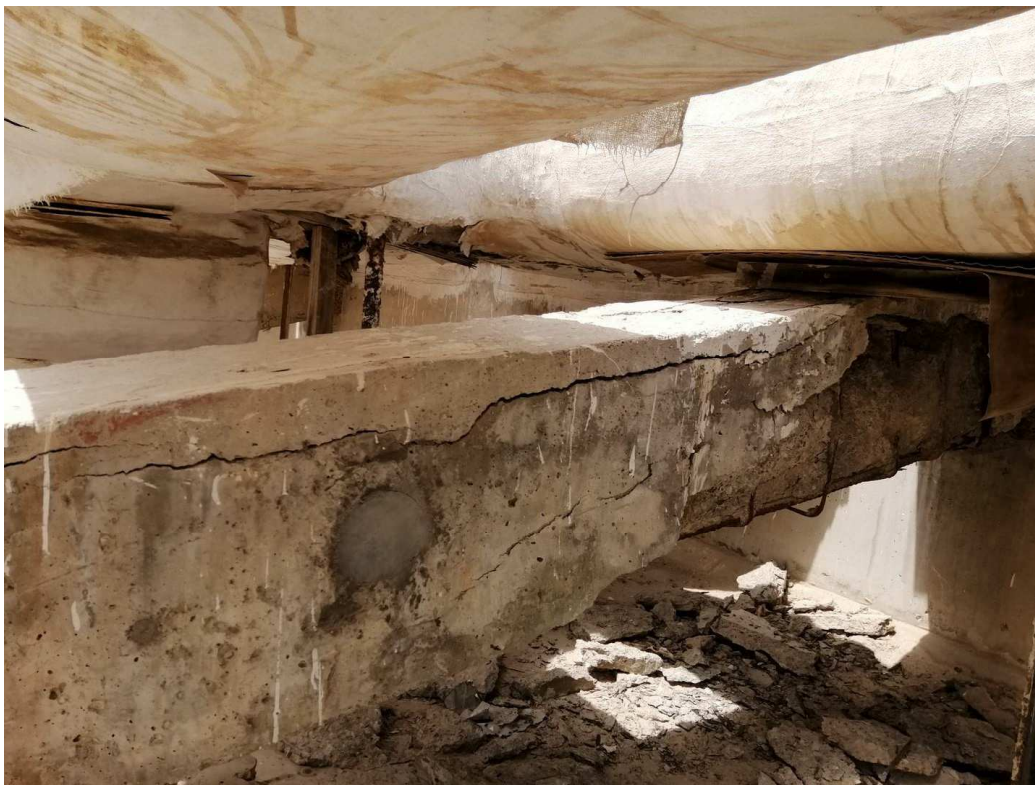
Figure 4-3 spalled cover and corroded steel at the playing area roof
