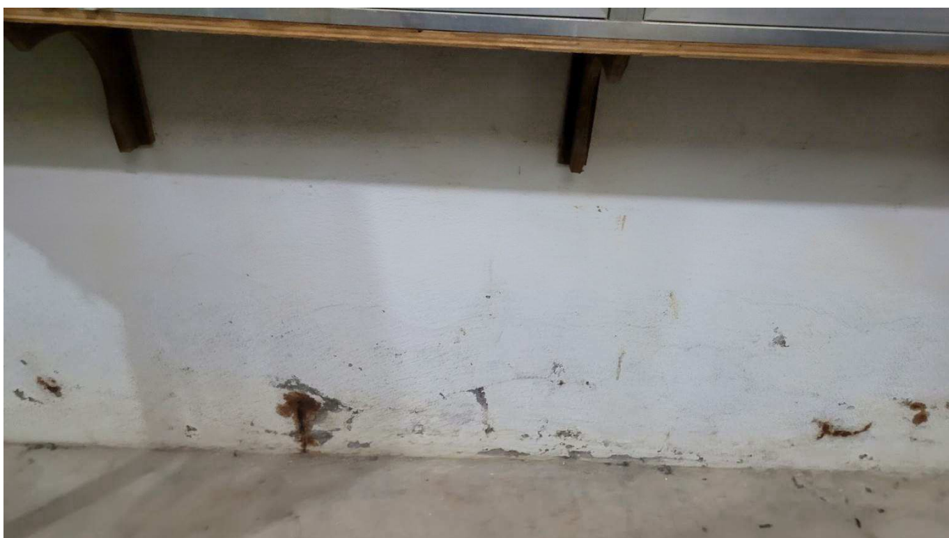
Figure 4-58 Delamination of the concrete cover and previous leakage in concrete wall
