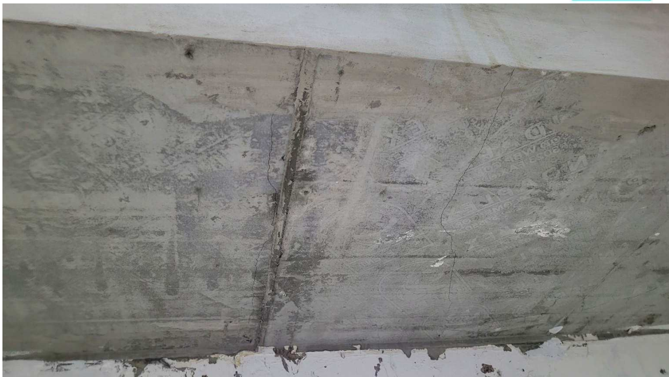
Figure 4-53 cracks in stands soffit
