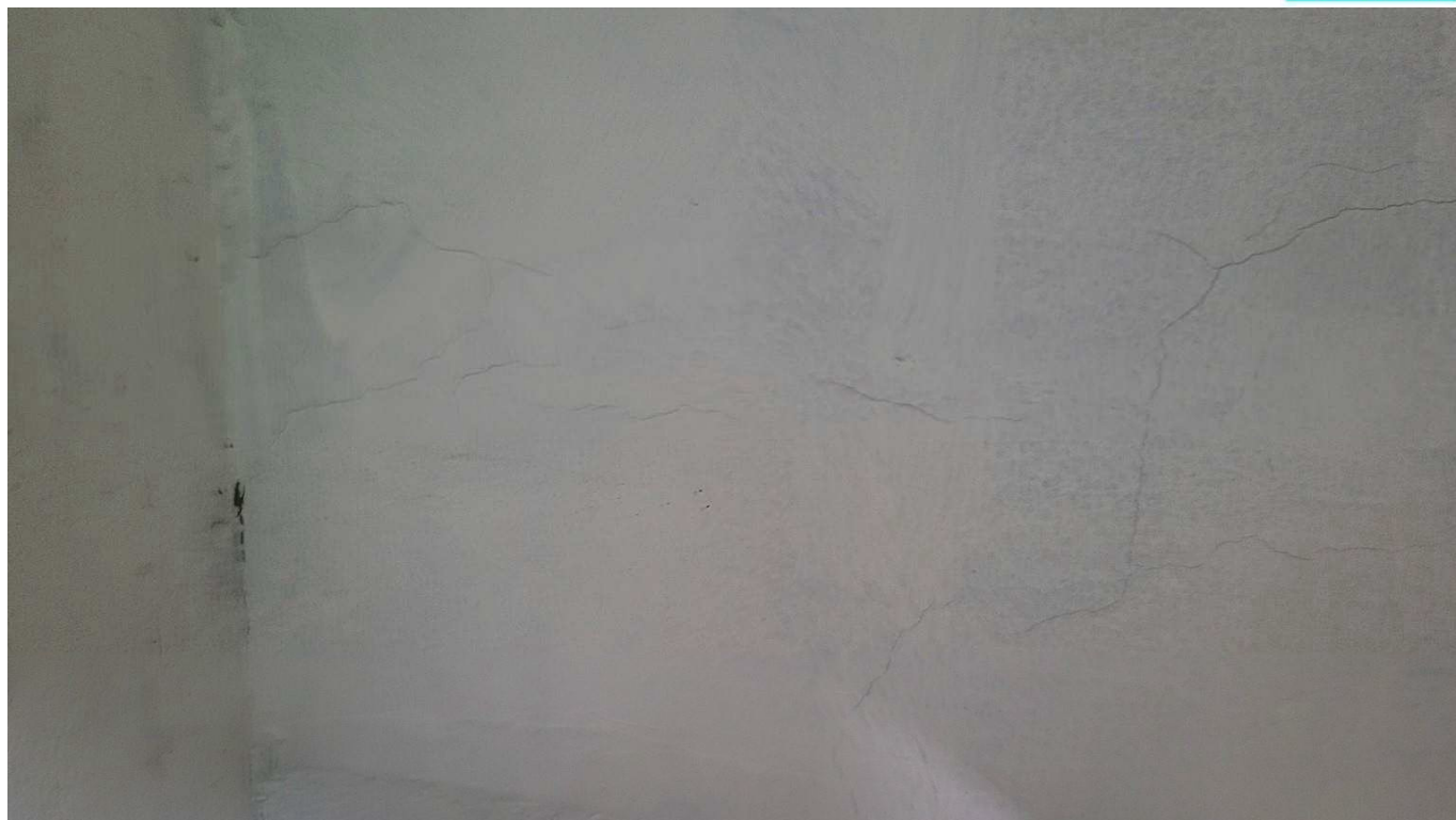
Figure 4-65 Crack in stands soffit
