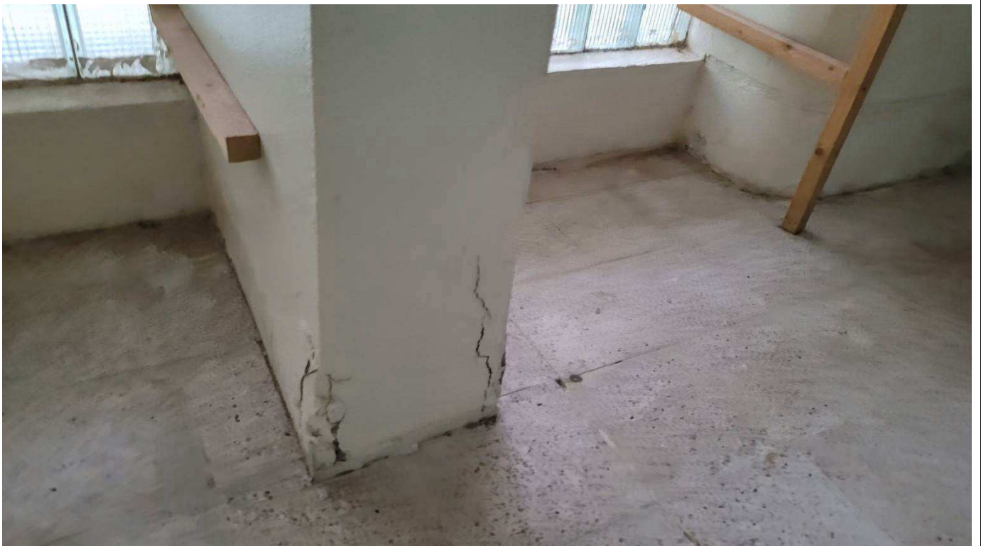
Figure 4-38 delamination in column
