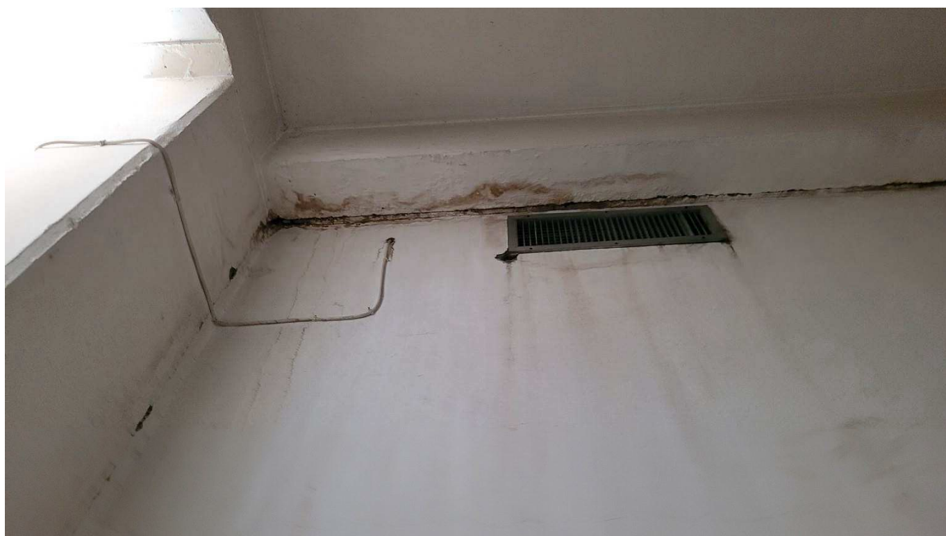
Figure 4-80 Previous leakage at expansion joint
