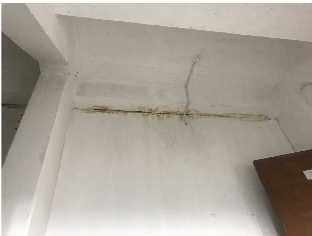
Figure 4-31 sign of previous leakage
