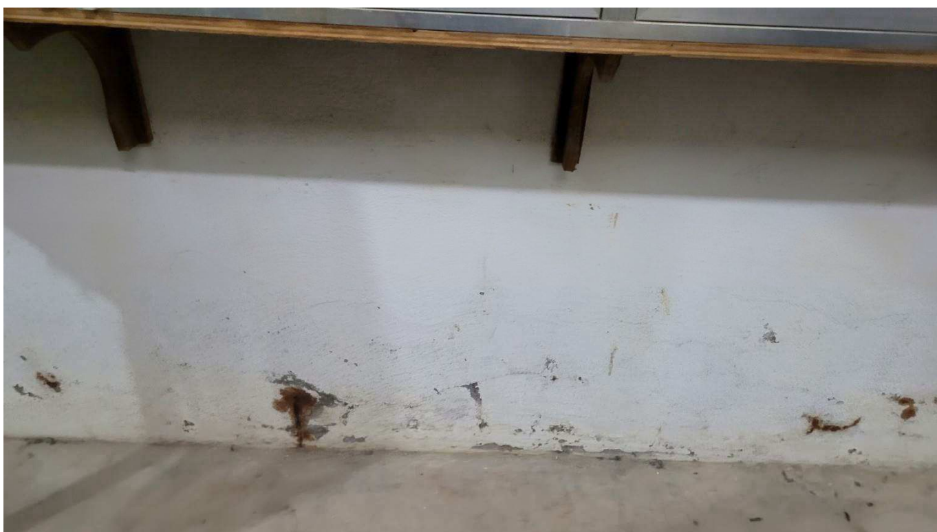
Figure 4-58 Delamination and previous leakage in concrete wall
