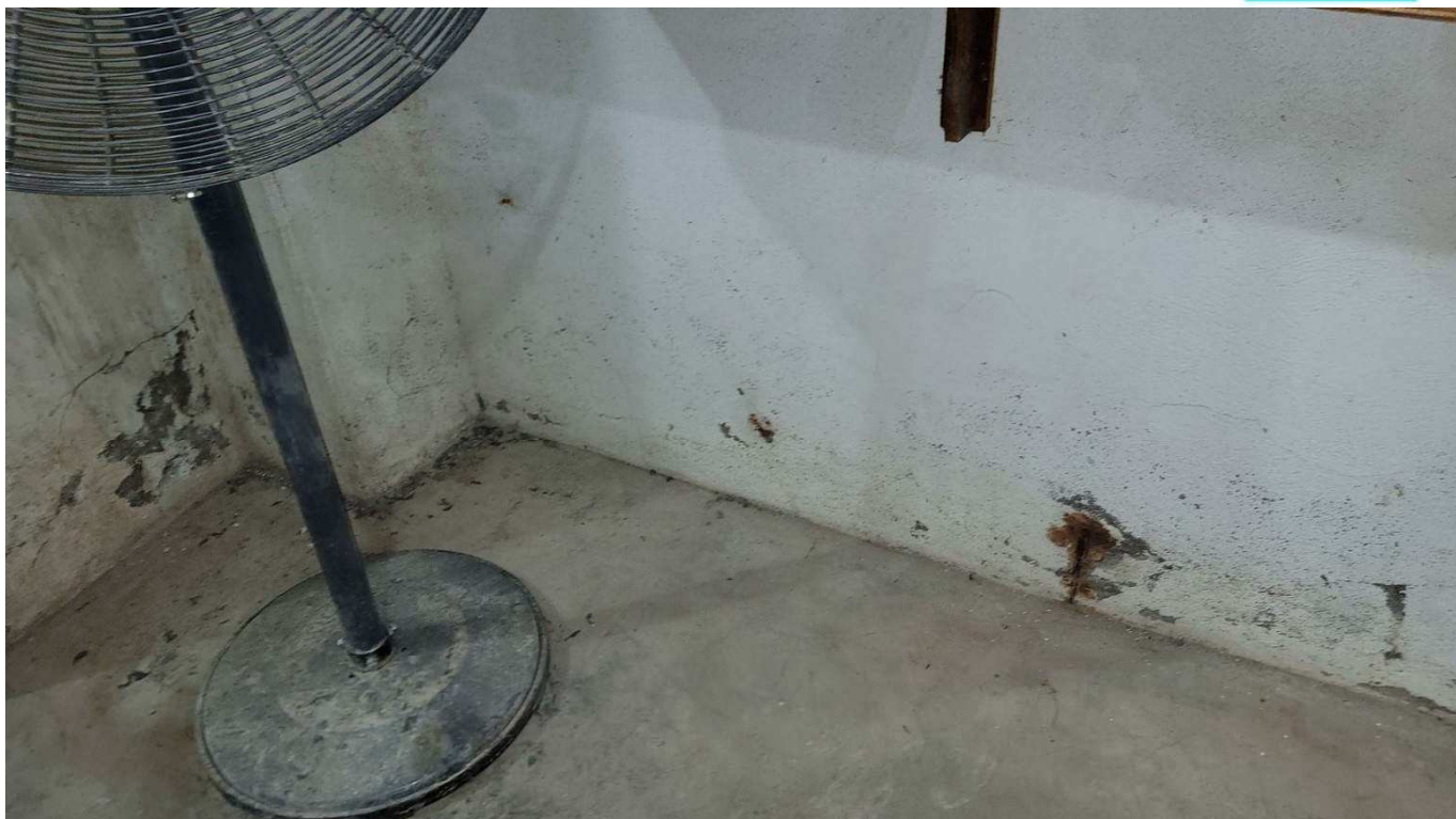
Figure 4-59 Delamination of the concrete cover and previous leakage in concrete wall
