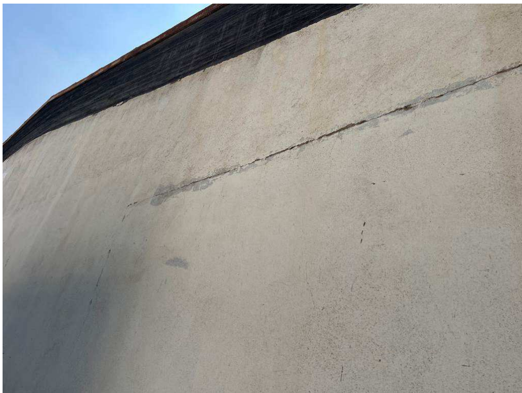
Figure 4-23 Crack between block wall and concrete element
