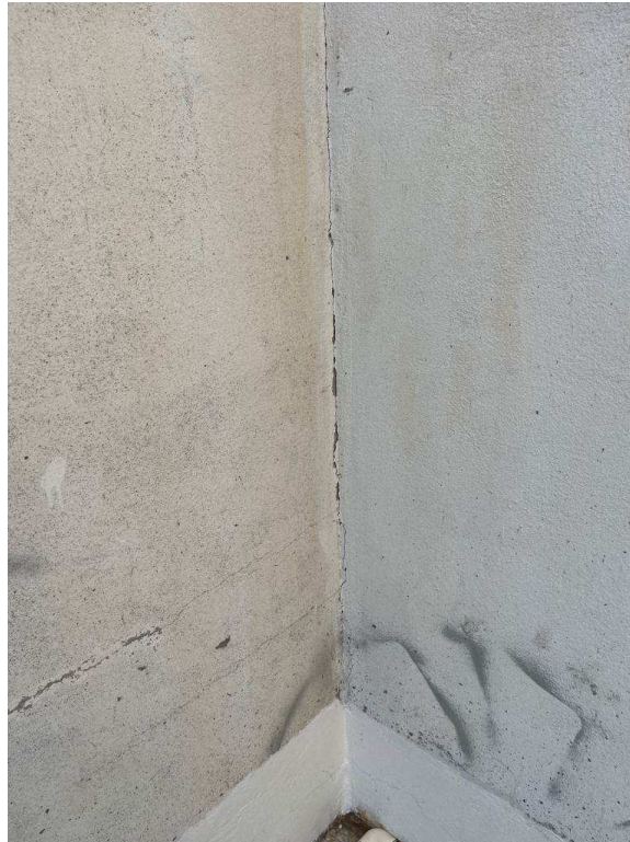
Figure 4-19 Cracks between block walls
