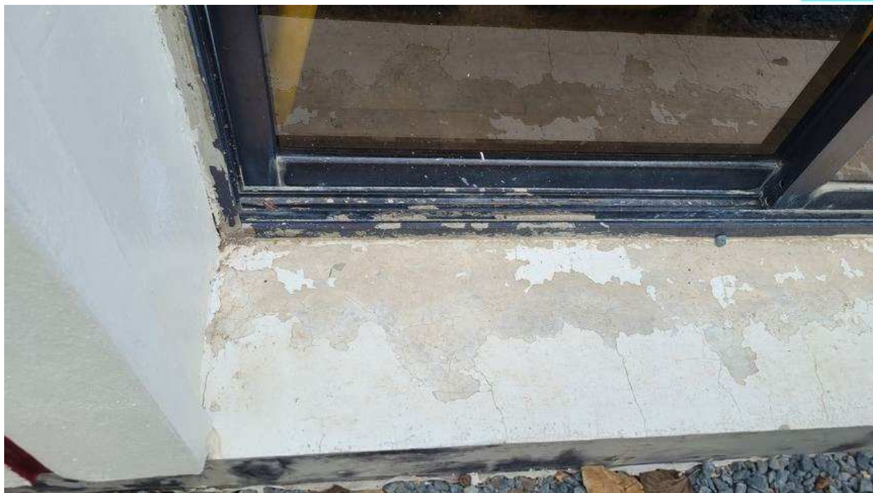
Figure 4-3 Dampness and cracks in ground beam
