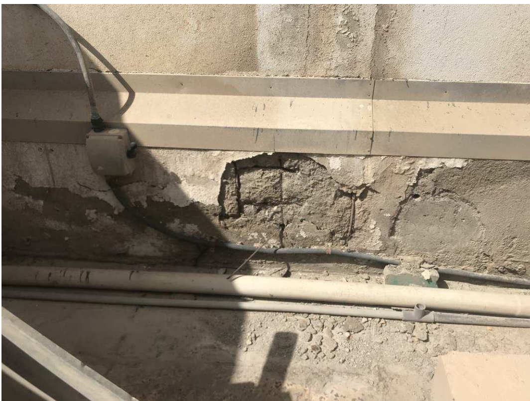
Figure 4-50 delamination and corrosion
