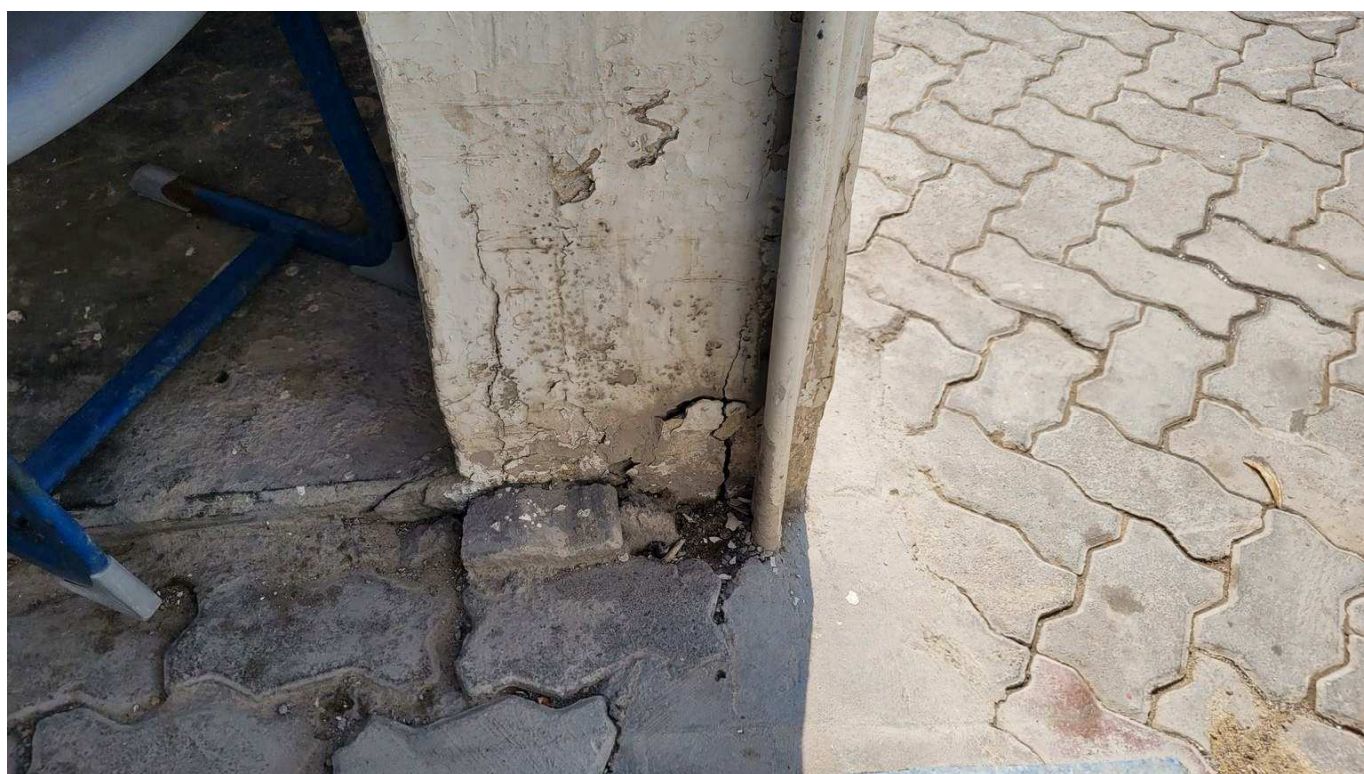
Figure 4-50 Delamination of the concrete cover and previous leakage in column
