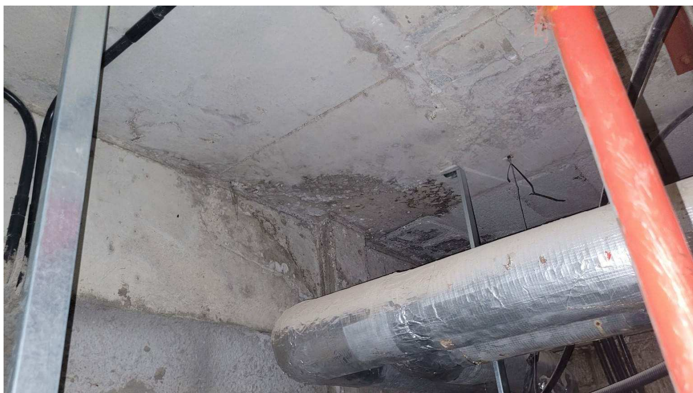
Figure 4-16 Previous leakage in beam and slab
