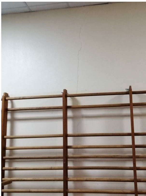
Figure 4-59 Cracks in Block wall
