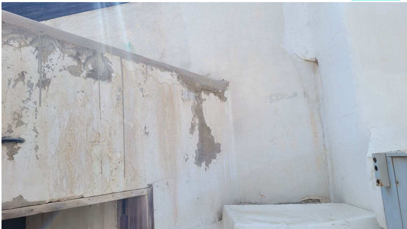
Figure 4-17 Previous leakage and cracks in roof walls and ceiling
