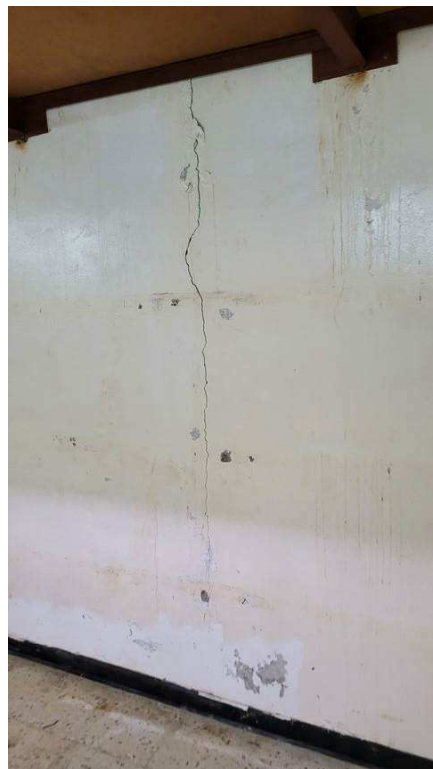
Figure 4-40 Dampness and cracks in block walls
