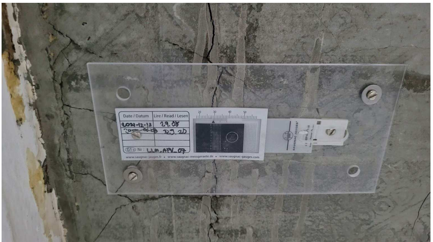
Figure 4-52 cracks and delamination in concrete wall below stands
