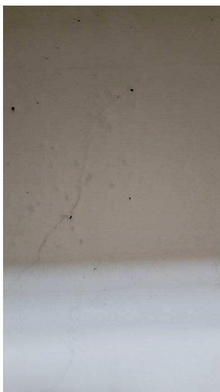
Figure 4-70 Cracks in stands soffit
