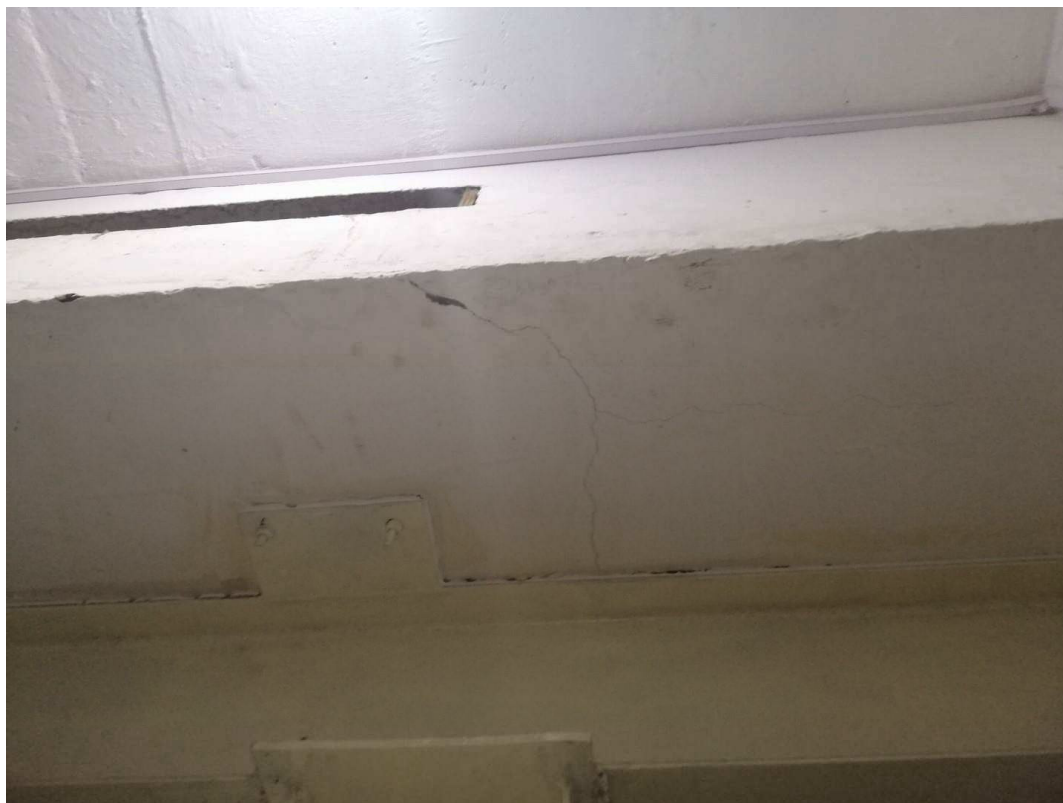
Figure 4-57 Cracks in stands
