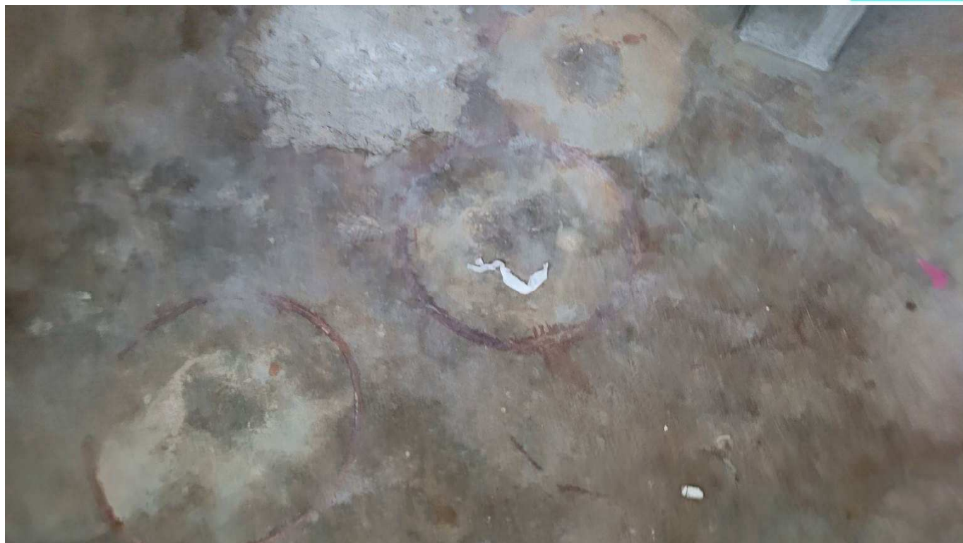
Figure 4-73 Sign of previous leakage in flooring
