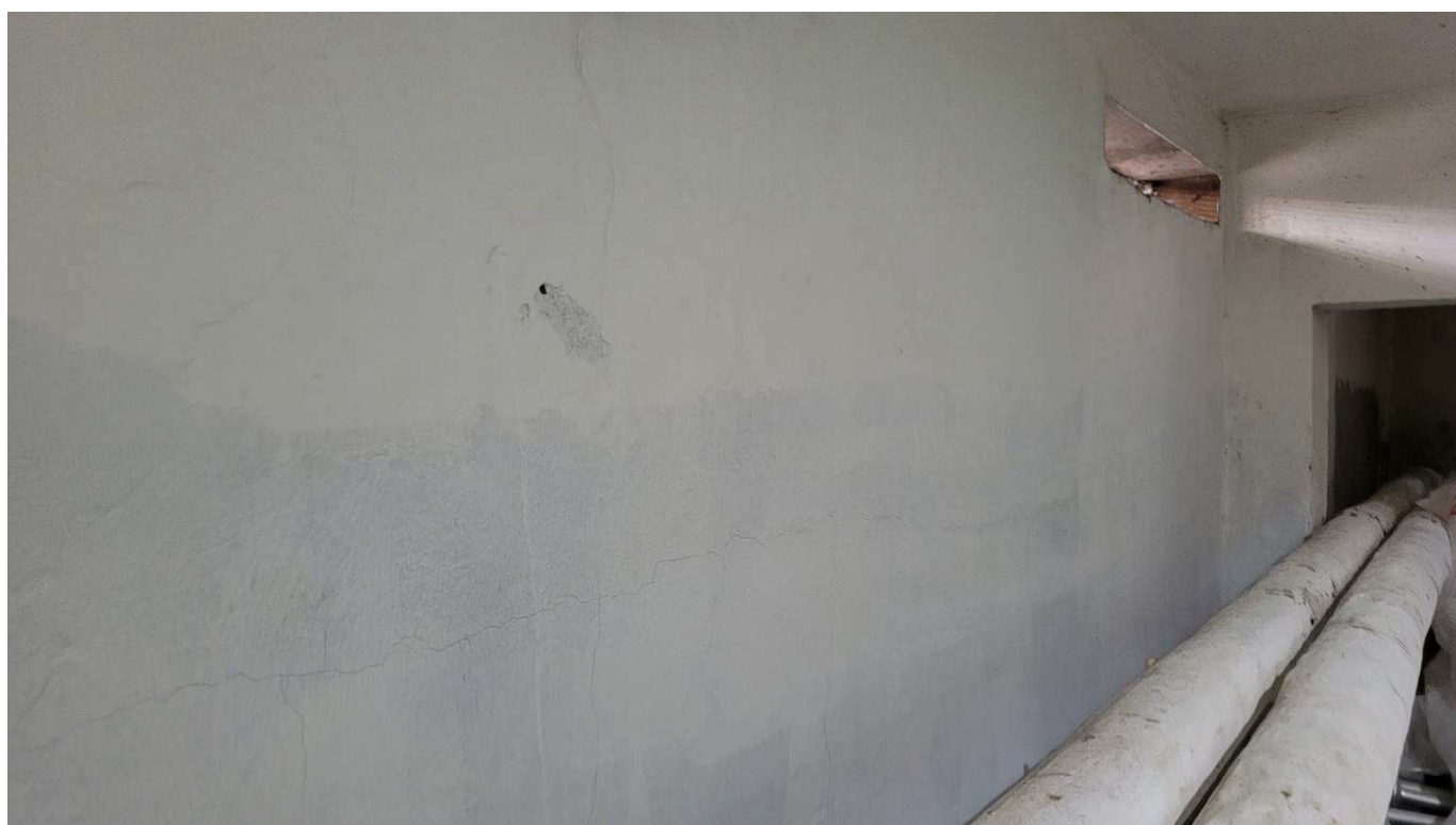
Figure 4-64 Crack in concrete wall
