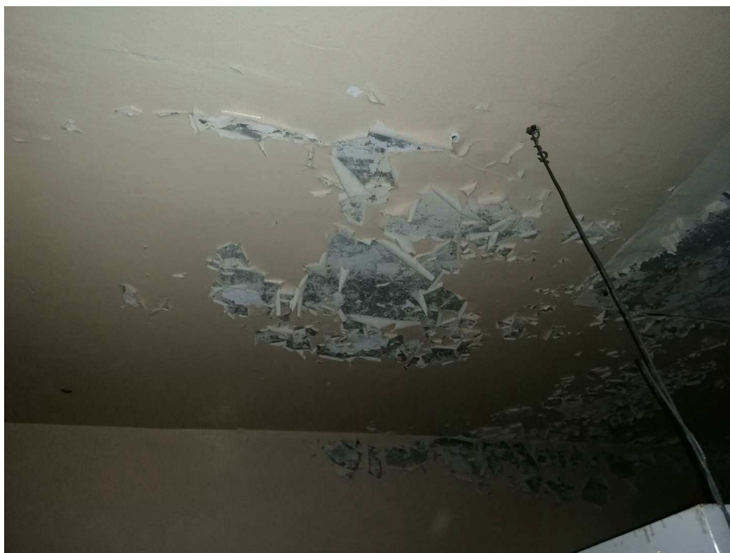
Figure 4-21 Previous dampness in slab
