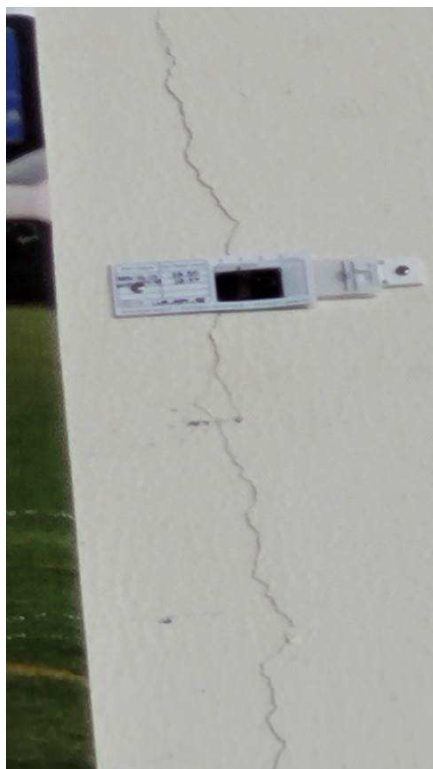
Figure 4-49 Crack in concrete wall
