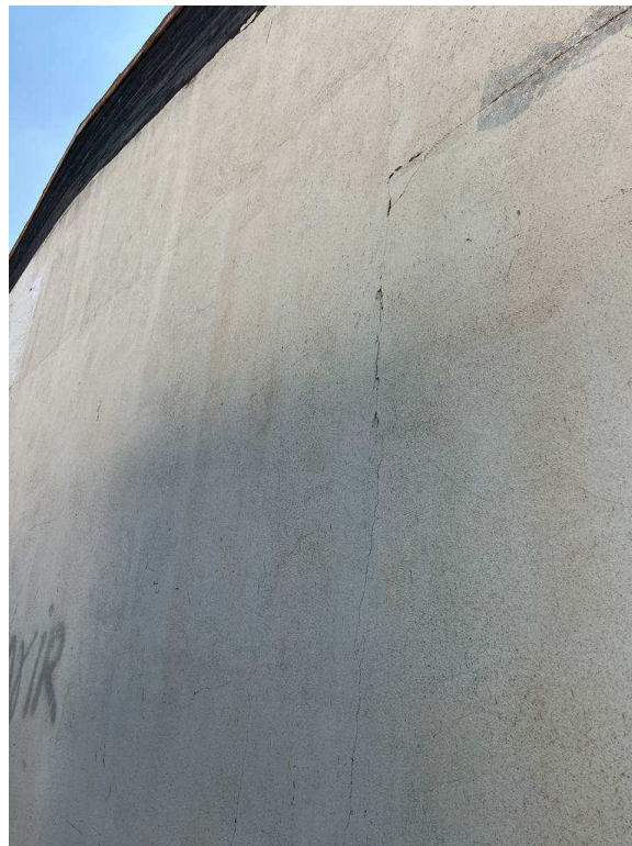
Figure 4-22 Dampness in block wall
