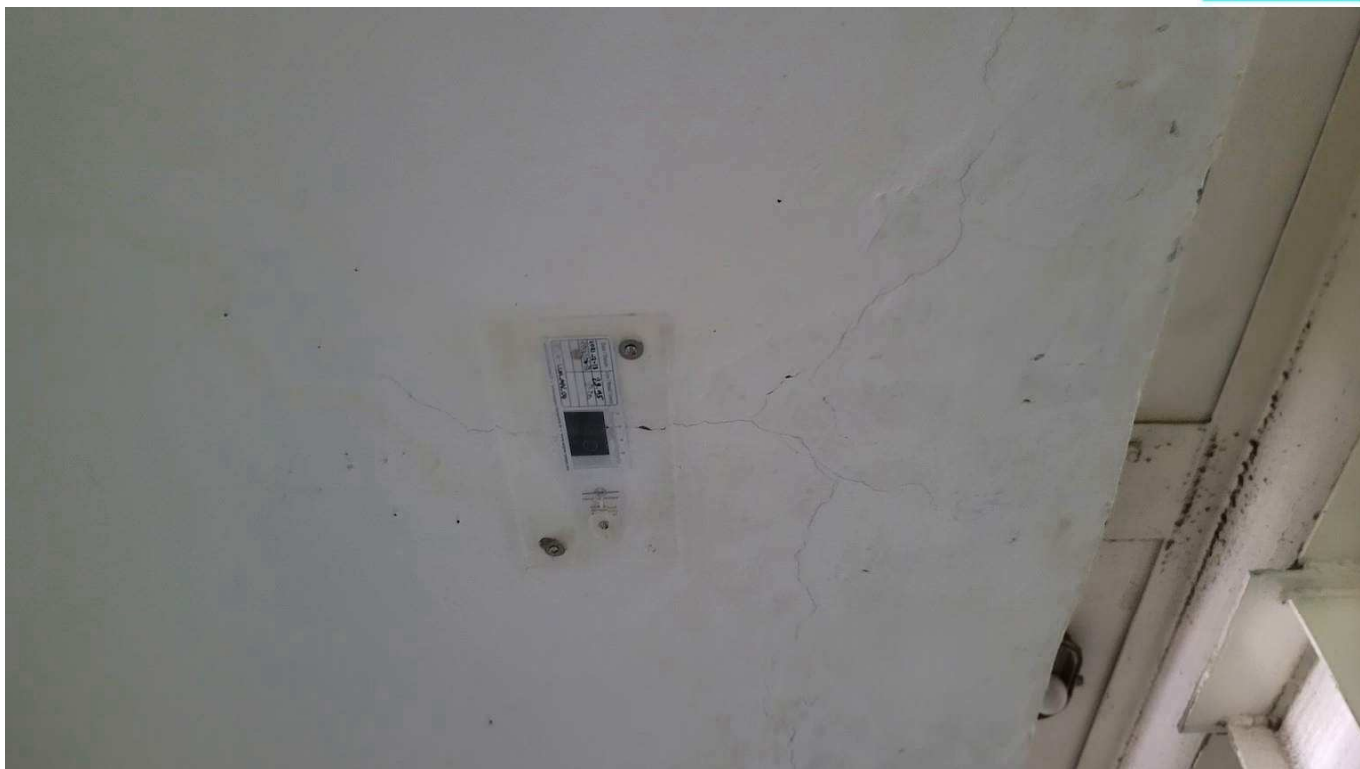
Figure 4-61 cracks in stands soffit
