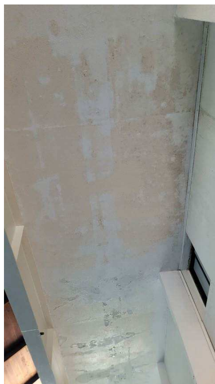
Figure 4-86 Previous leakage in slab soffit
