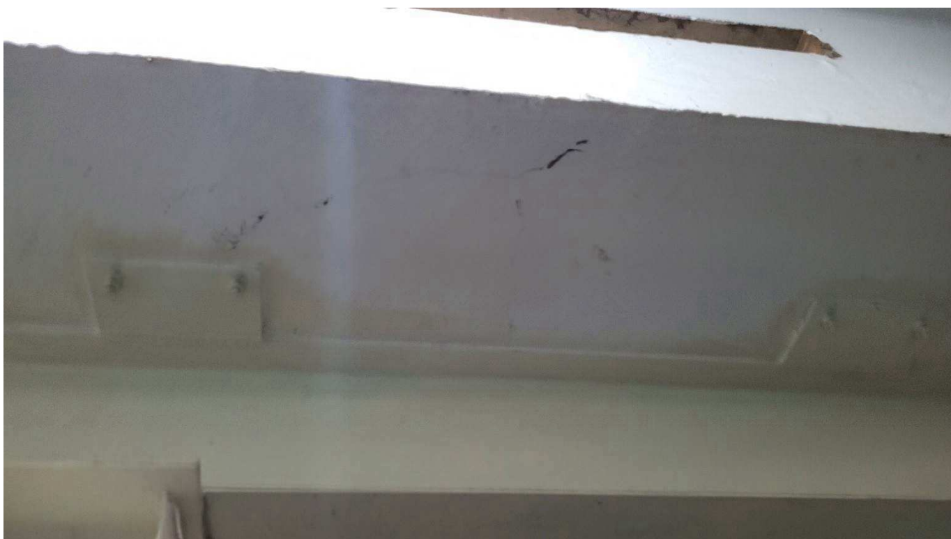
Figure 4-66 Crack in stands soffit
