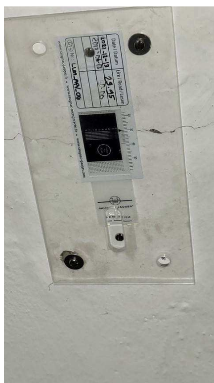
Figure 4-60 Cracks in concrete below stands
