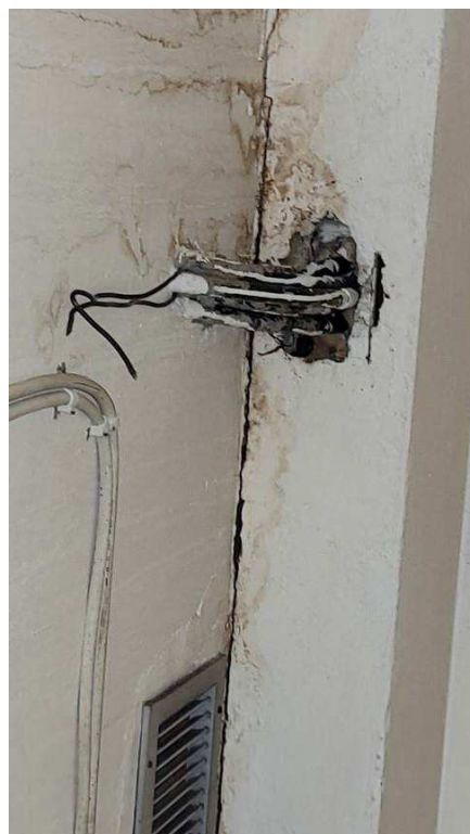
Figure 4-76 Previous leakage in expansion joint
