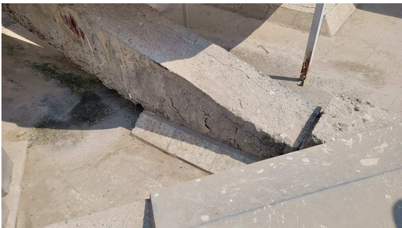
Figure 4-30 Delamination of the concrete cover in roof beam
