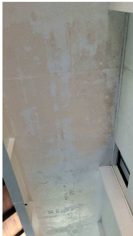
Figure 4-86 Previous leakage in slab soffit
