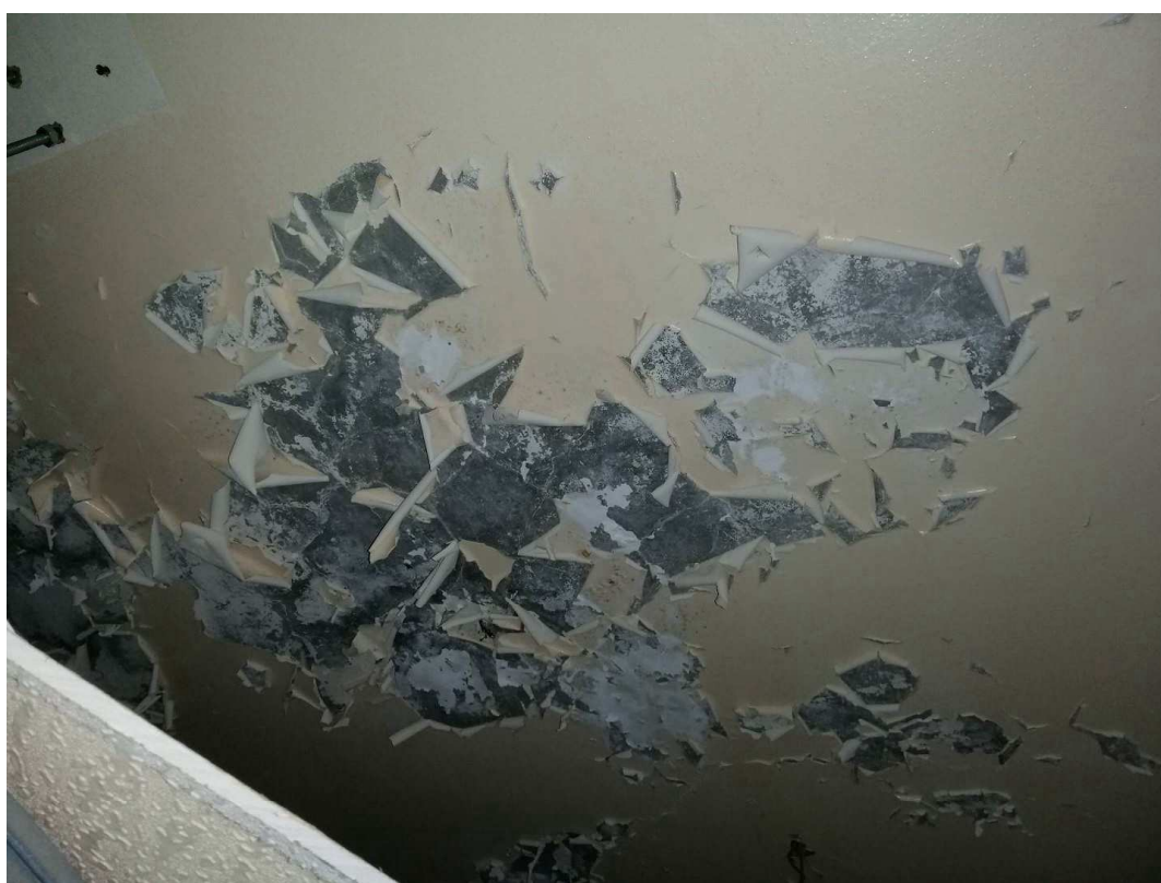
Figure 4-22 previous dampness in slab
