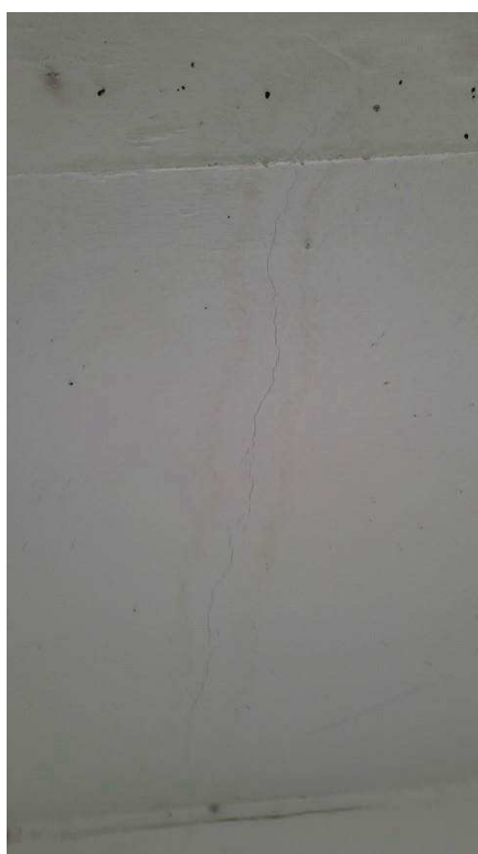
Figure 4-62 crack with previous leakage in stands soffit
