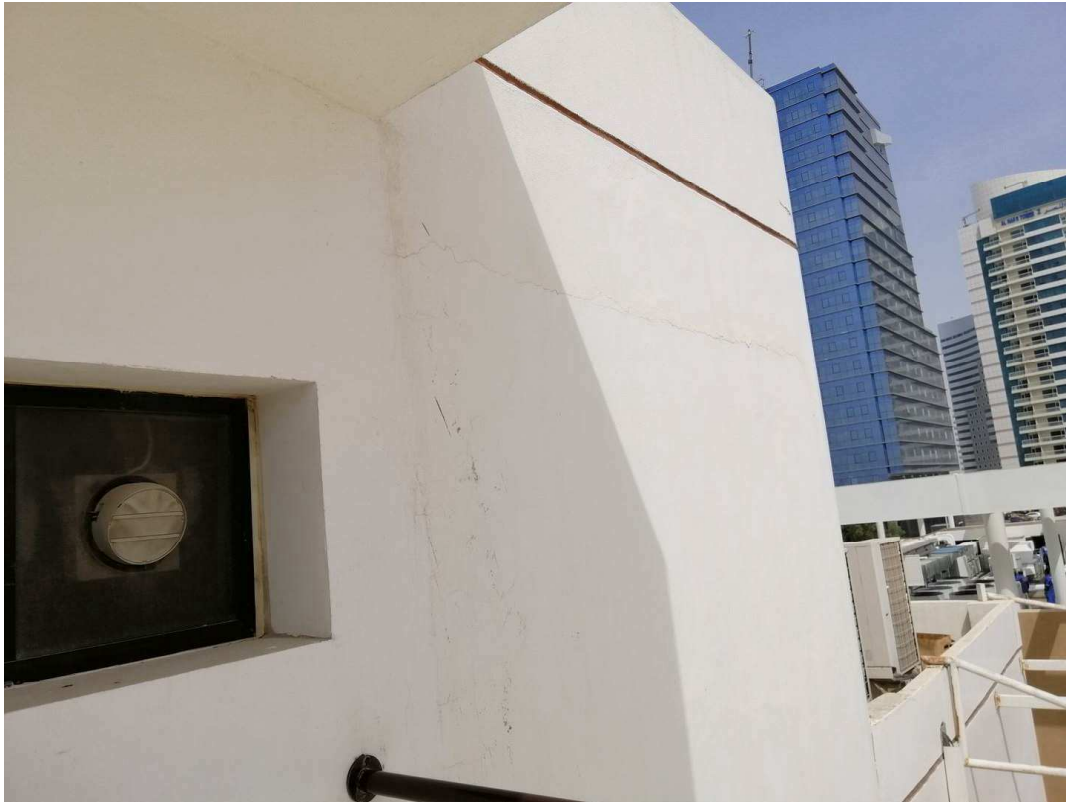
Figure 4-25 crack between block wall and concrete element
