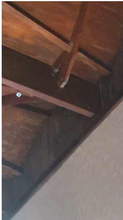
Figure 4-91 previous leakage in wooden slab soffit
