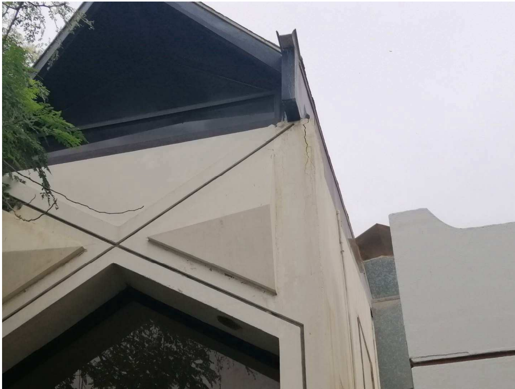
Figure 4-14 Cracks in column due to steel corrosion
