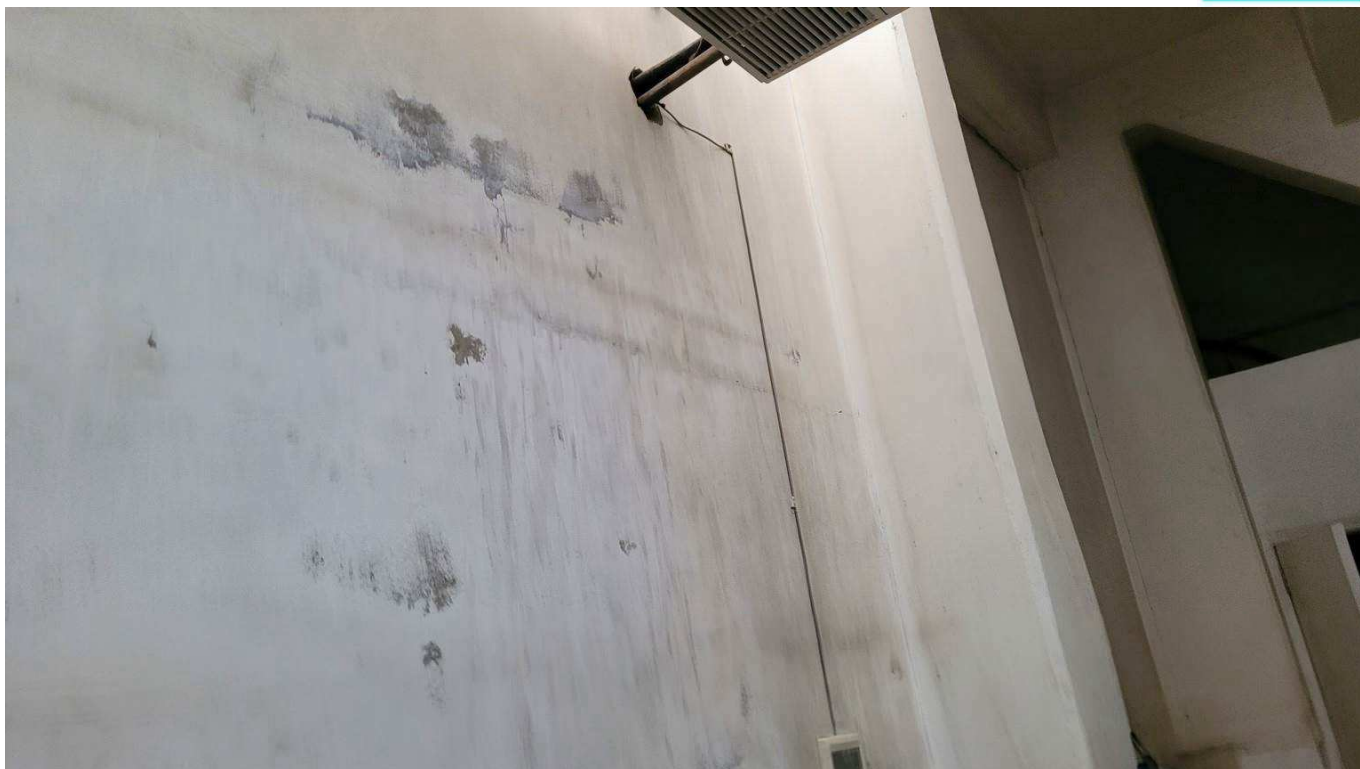
Figure 4-81 Dampness and cracks in block wall
