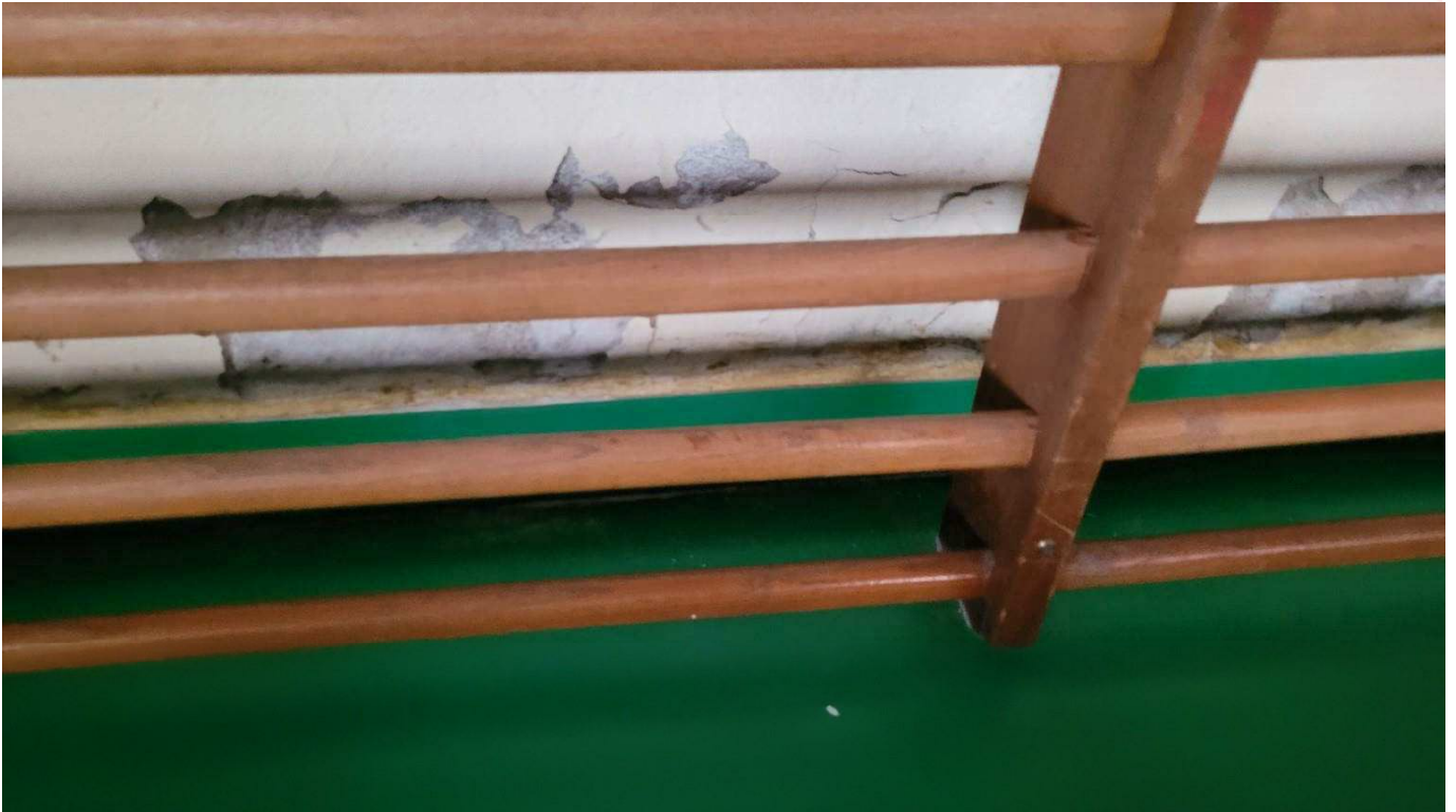
Figure 4-45 Dampness and Delamination of the concrete cover in ground beam
