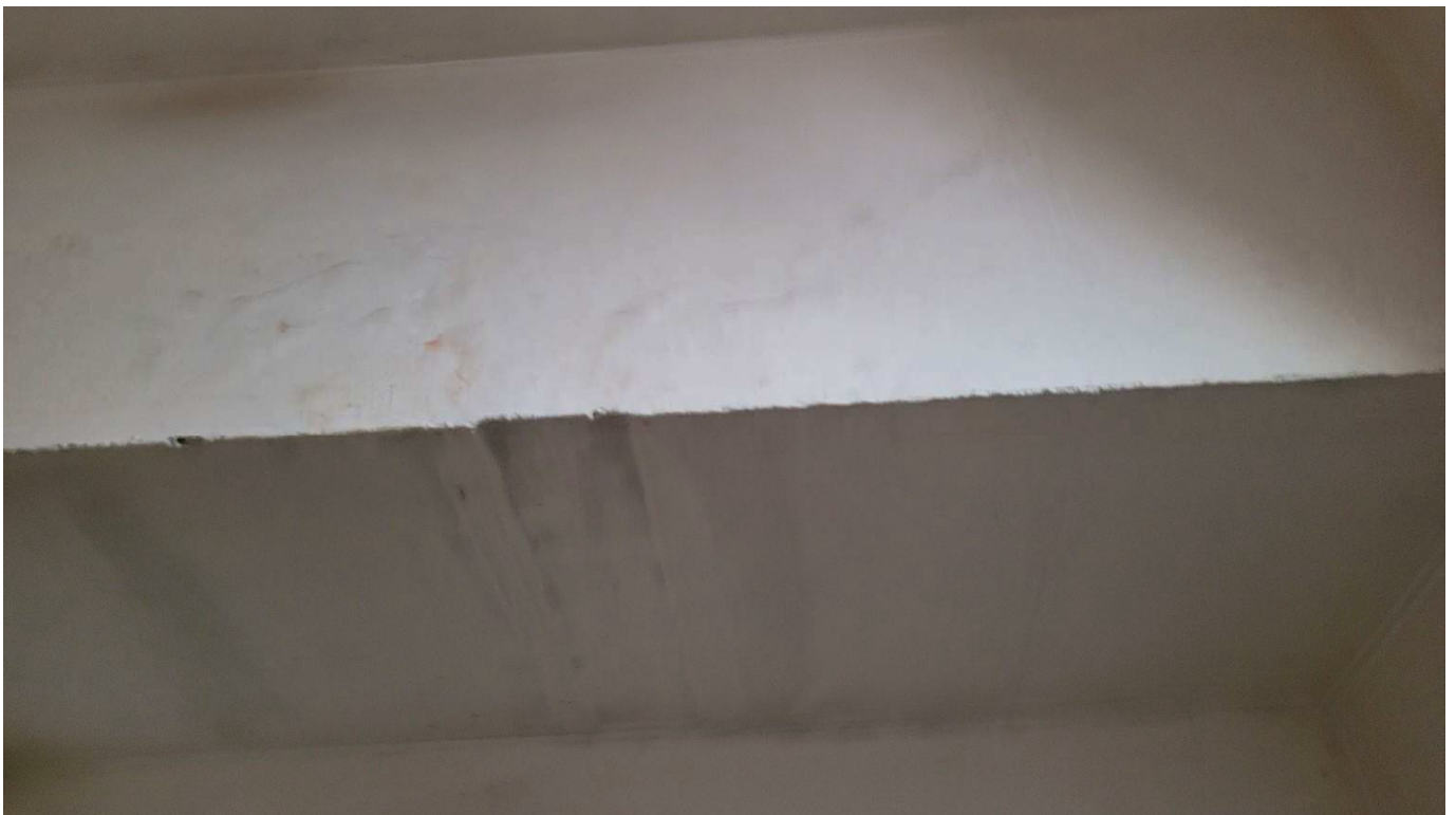
Figure 4-68 previous leakage in stands soffit
