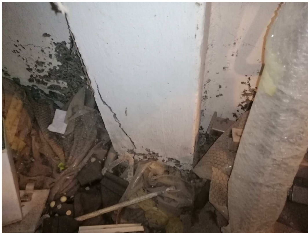
Figure 4-55 Cracks in column
