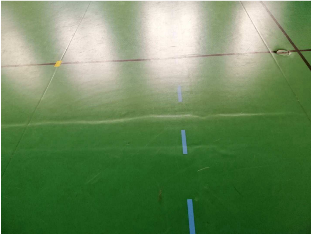
Figure 4-63 bulging in the floor
