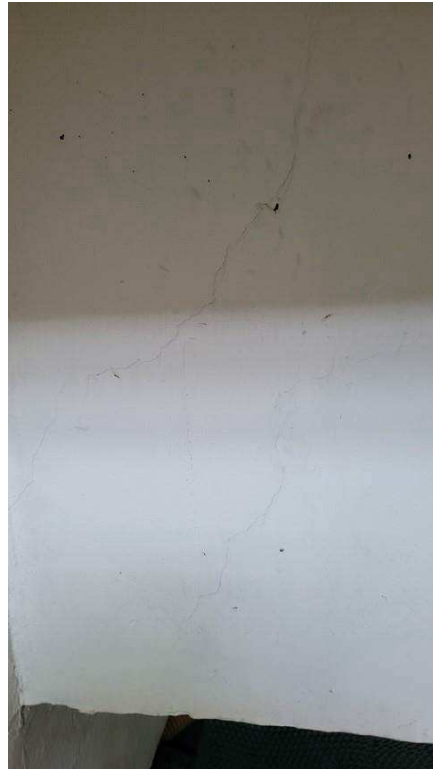
Figure 4-69 cracks in stands soffit
