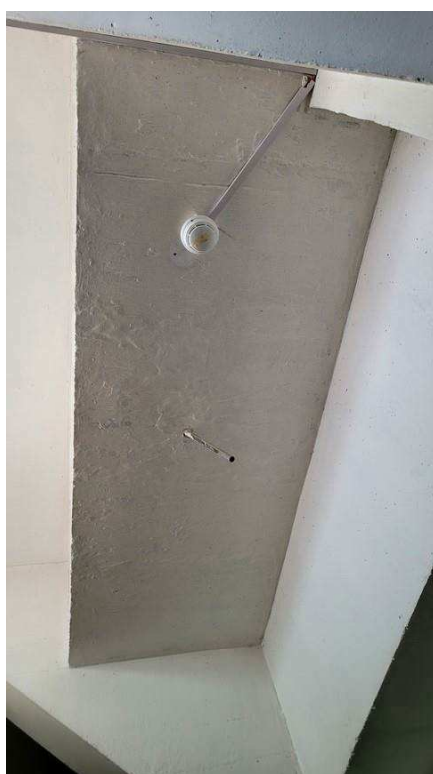
Figure 4-82 Previous leakage in the stand's soffit
