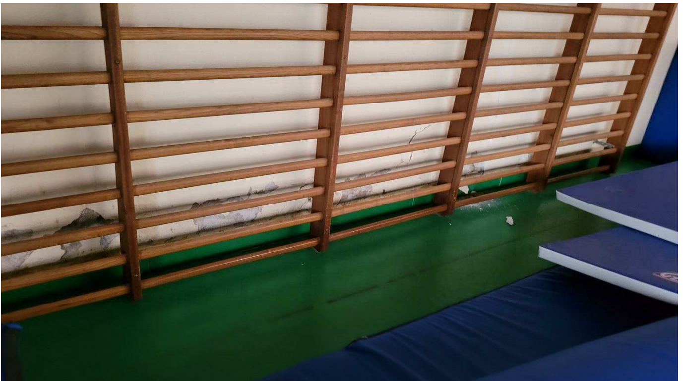
Figure 4-46 Dampness and Delamination of the concrete cover in ground beam
