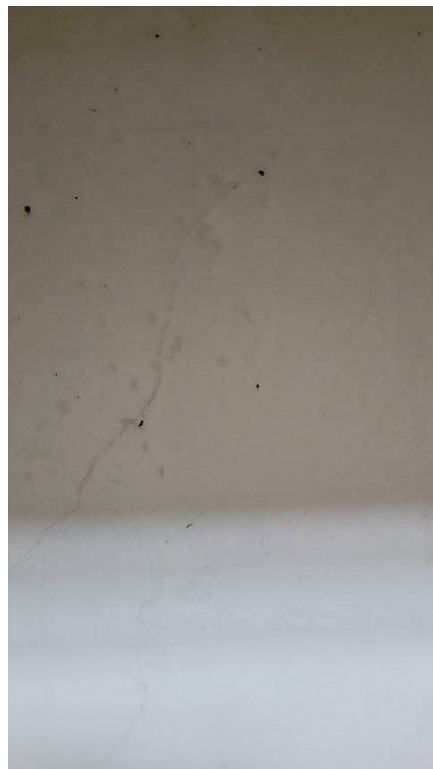
Figure 4-70 cracks in stands soffit
