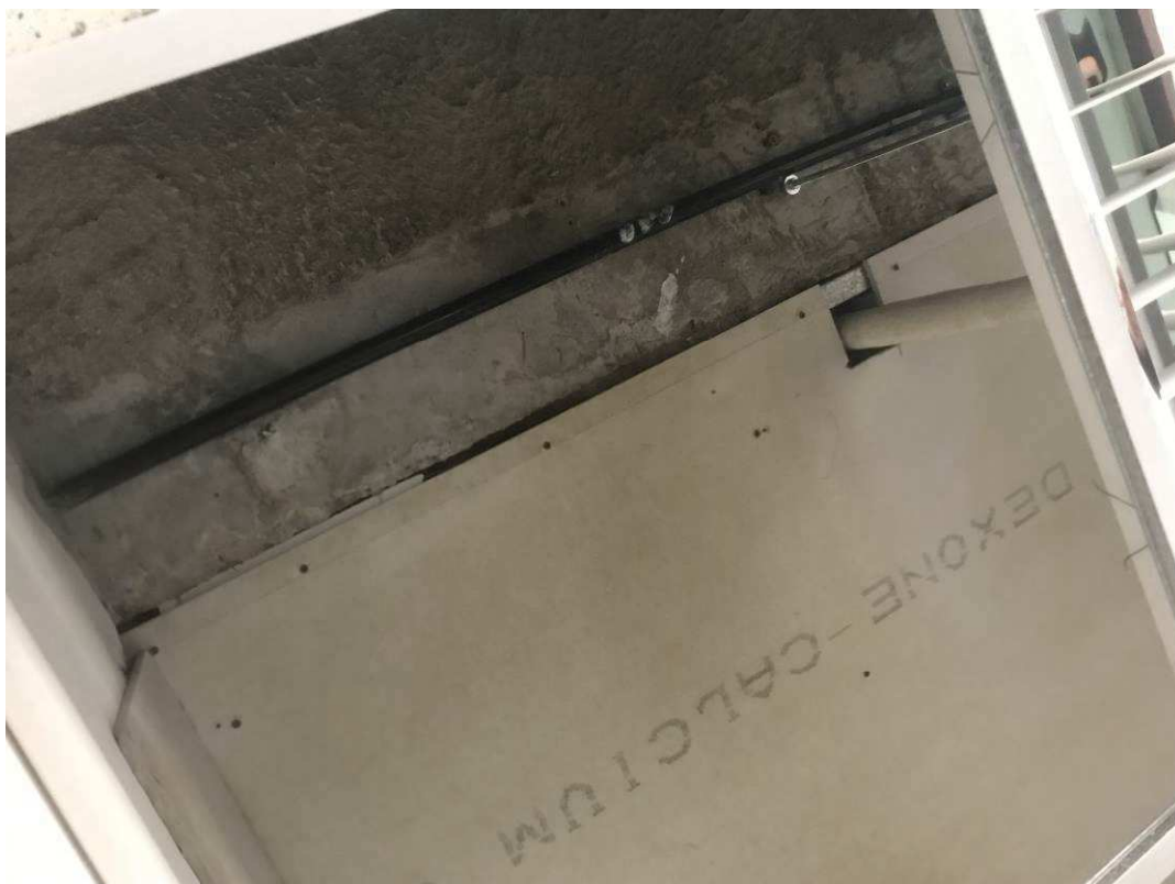
Figure 4-24 slab opening which not closed properly
