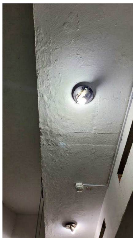
Figure 4-54 Previous leakage in stands soffit
