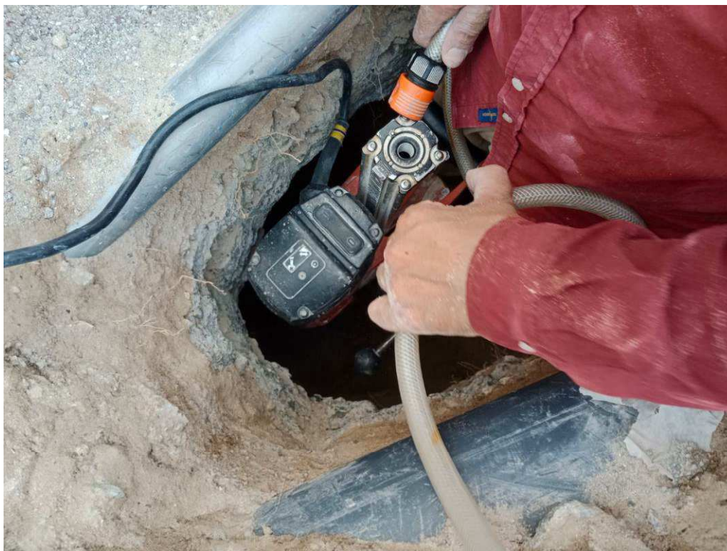
Figure 4-92 During coring the foundation
