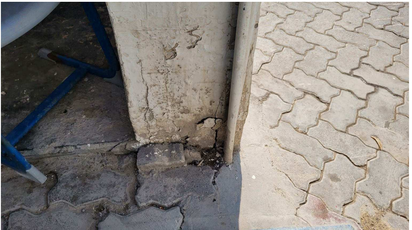
Figure 4-50 delamination and previous leakage in column
