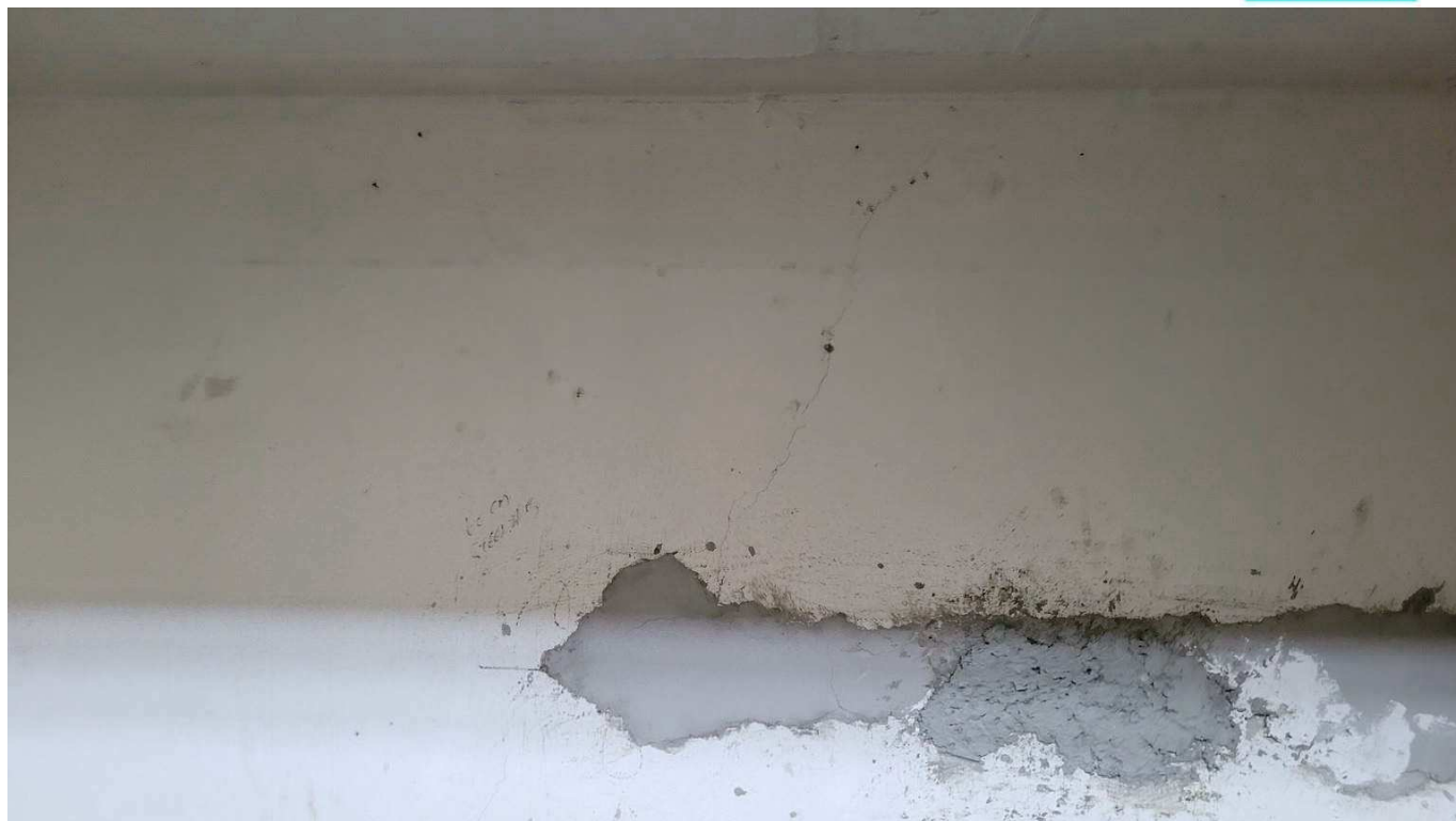
Figure 4-71 Cracks in stands soffit
