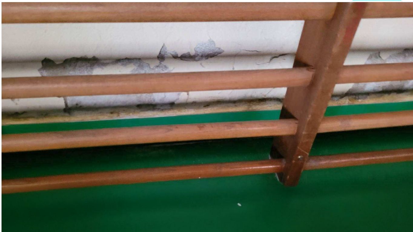
Figure 4-45 Dampness and delamination in ground beam
