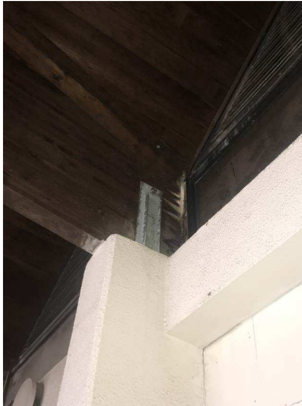
Figure 4-46 Dampness in wooden beam
