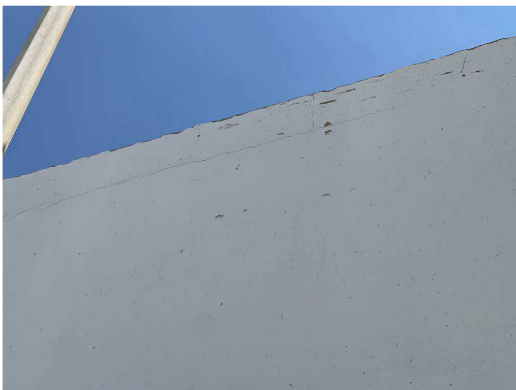
Figure 4-24 Crack between block wall and slab
