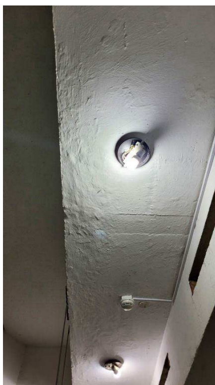
Figure 4-54 previous leakage in stands soffit
