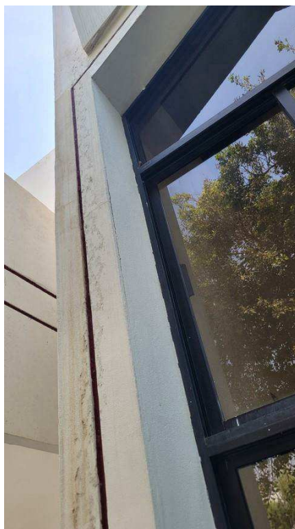
Figure 4-4 previous leakage in column
