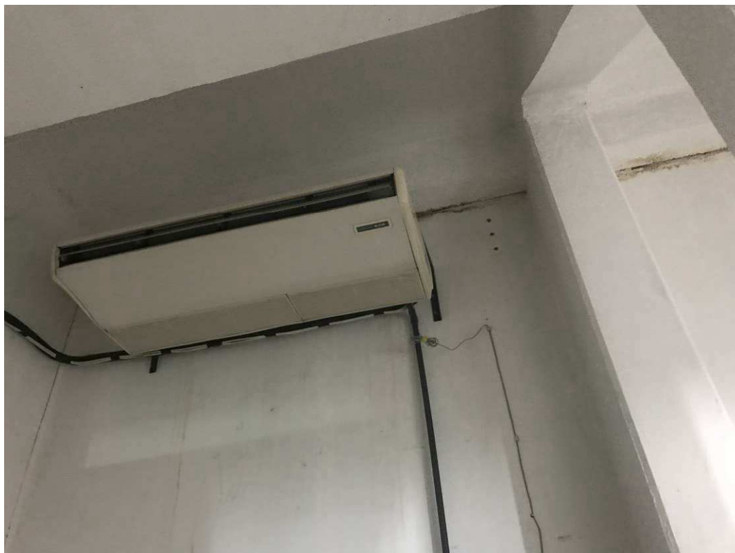
Figure 4-32 sign of previous leakage
