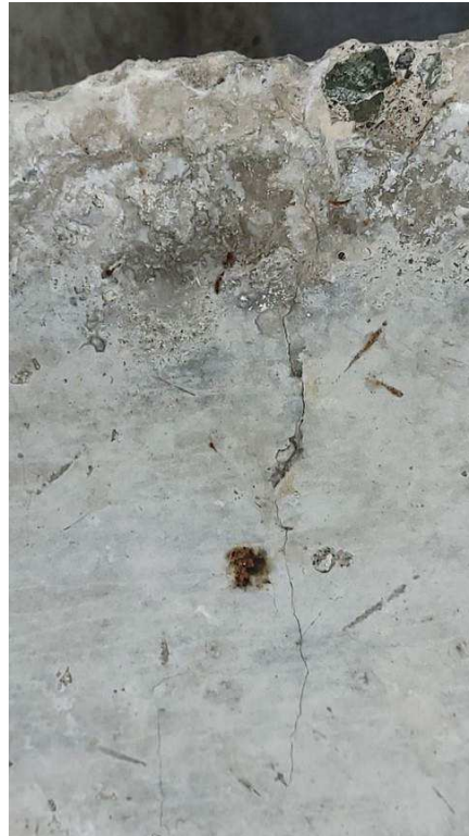
Figure 4-31 Crack in slab soffit
