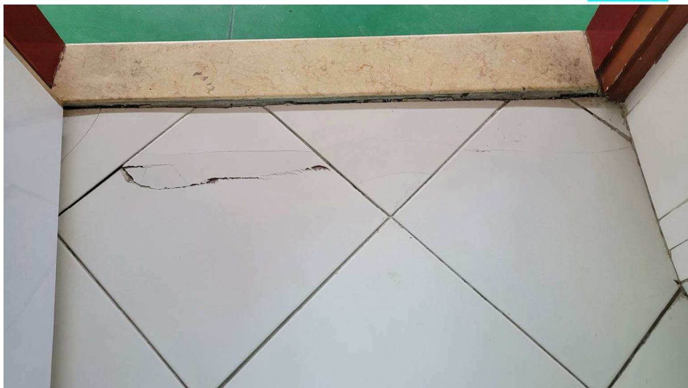
Figure 4-47 cracks in tiles in toilets in gym
