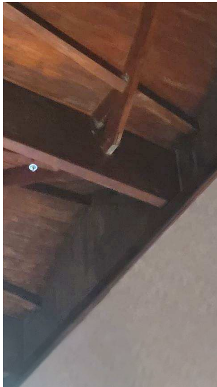
Figure 4-91 Previous leakage in wooden slab soffit
