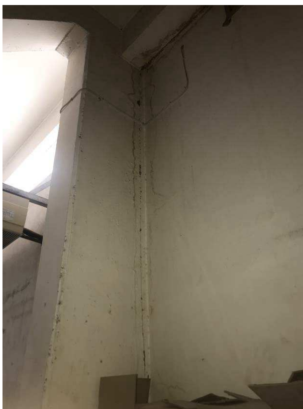
Figure 4-33 Crack between block wall and concrete element.
