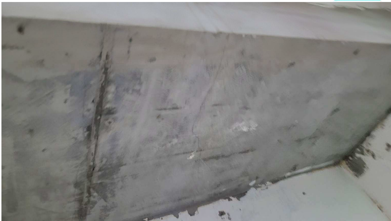
Figure 4-57 Cracks in the stand's soffit
