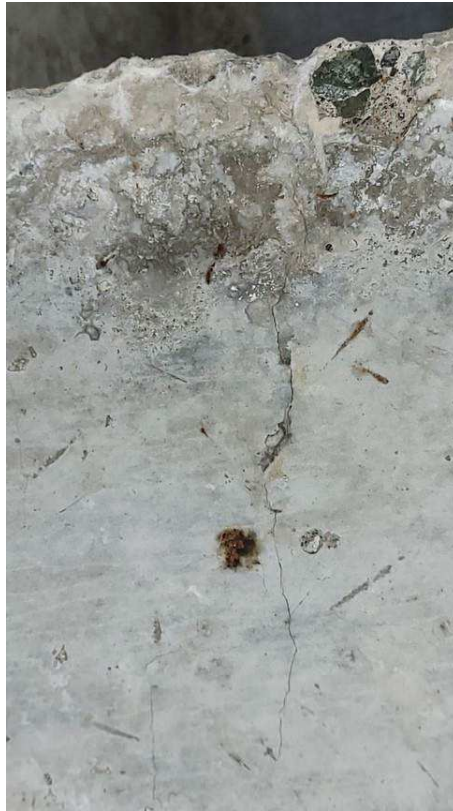
Figure 4-31 Crack in slab soffit
