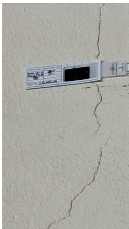
Figure 4-48 Crack in concrete wall
