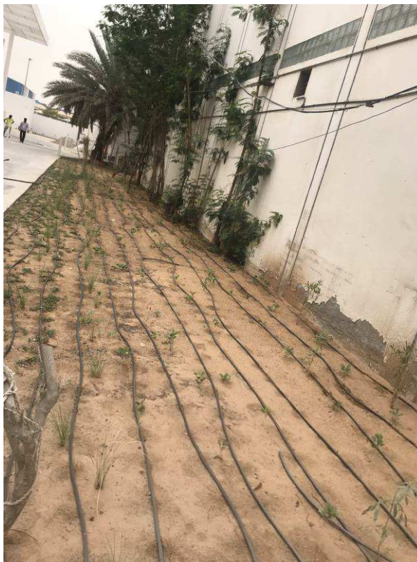
Figure 4-47 landscaping work touching the pool which affect the quality of concrete
