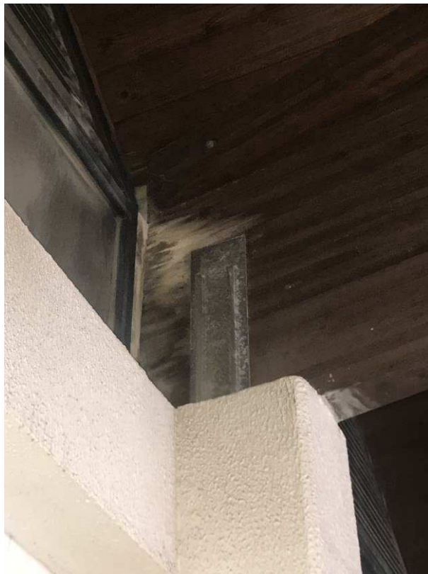
Figure 4-45 Dampness in wooden beam
