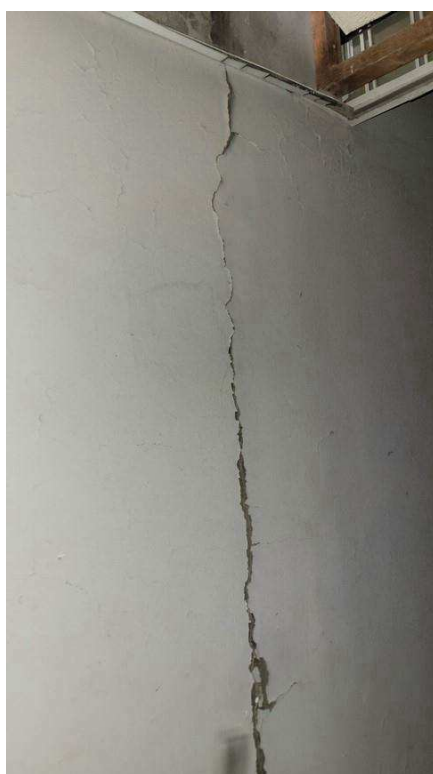
Figure 4-12 Crack between block wall and concrete element
