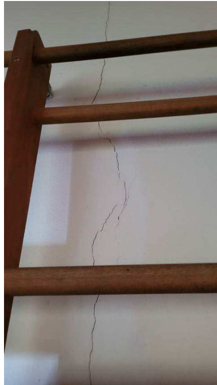
Figure 4-43 cracks in block wall
