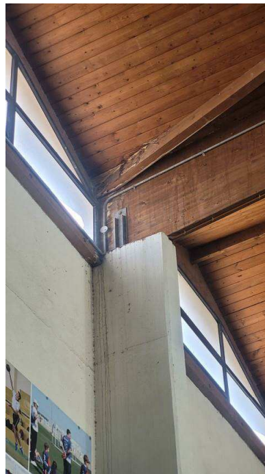
Figure 4-36 previous leakage in column and wooden roof
