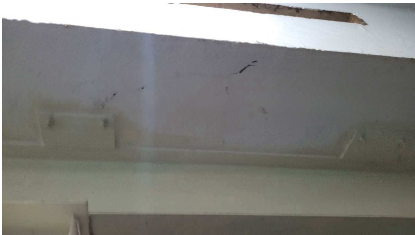
Figure 4-66 Crack in stands soffit
