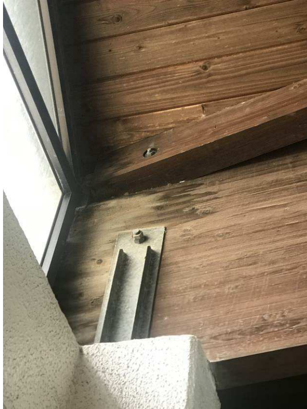
Figure 4-44 Dampness in wooden beam
