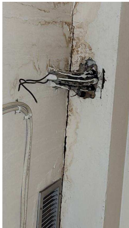
Figure 4-76 previous leakage in expansion joint
