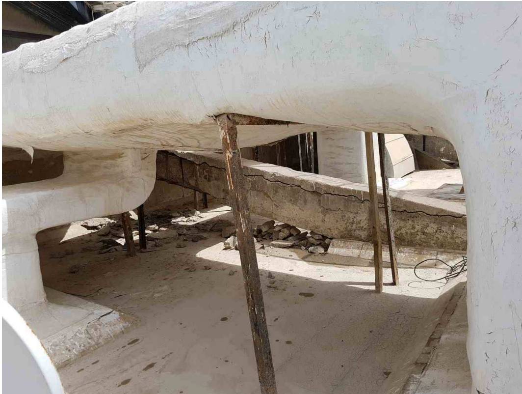
Figure 4-6 Cracks in beam due to steel reinforcement corrosion
