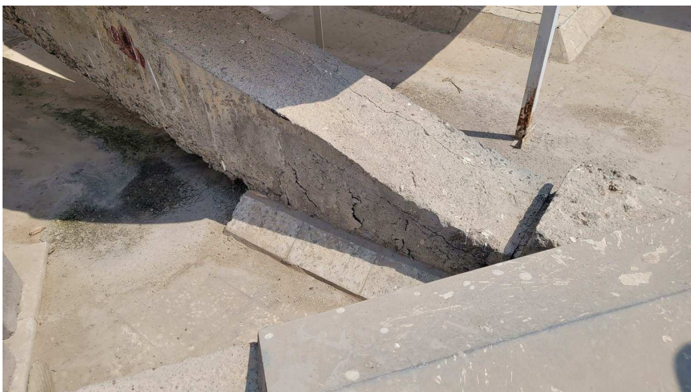
Figure 4-30 delamination in beam of the roof
