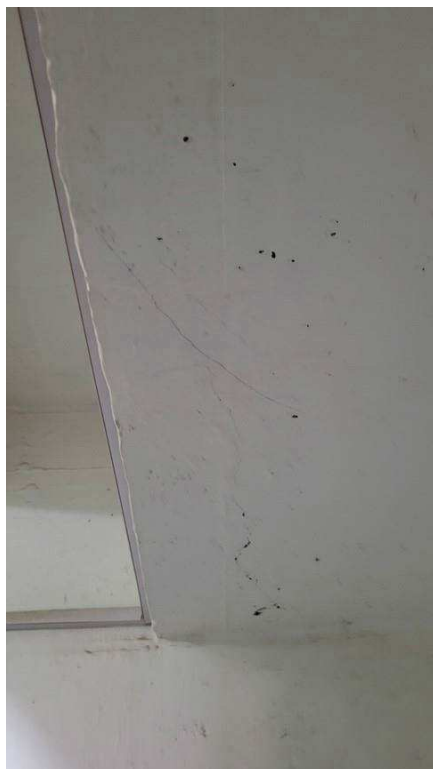
Figure 4-63 Crack in stands soffit
