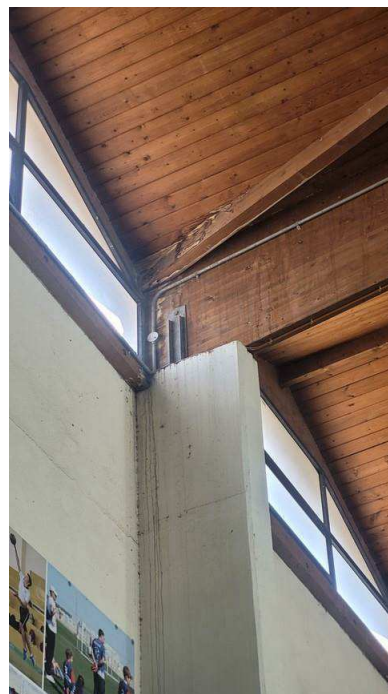
Figure 4-36 Previous leakage in column and wooden roof
