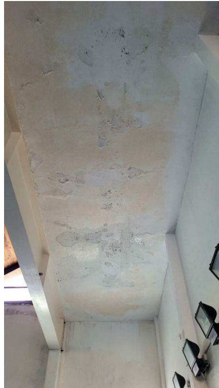
Figure 4-85 Previous leakage in slab soffit
