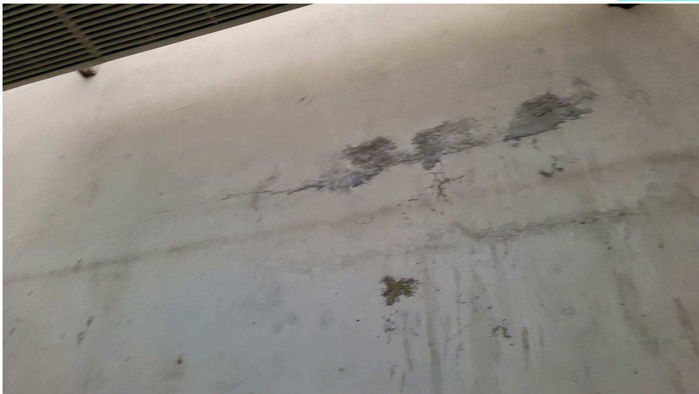
Figure 4-77 Cracks and dampness in wall
