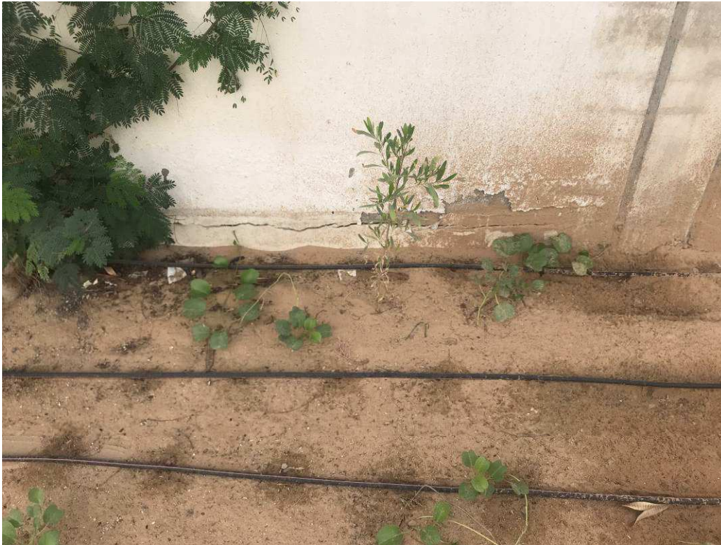
Figure 4-48 landscaping work touching the pool which affect the quality of concrete
