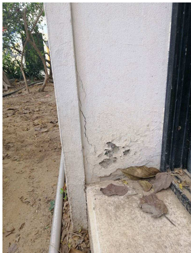
Figure 4-13 Cracks in column due to steel corrosion
