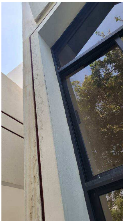
- Figure 4-4 previous leakage in column
