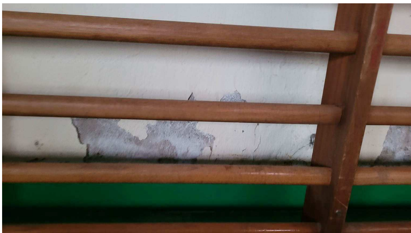
Figure 4-44 Dampness and Delamination of the concrete cover in ground beam
