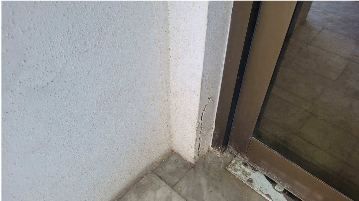
Figure 4-1 Delamination of the concrete cover in column
