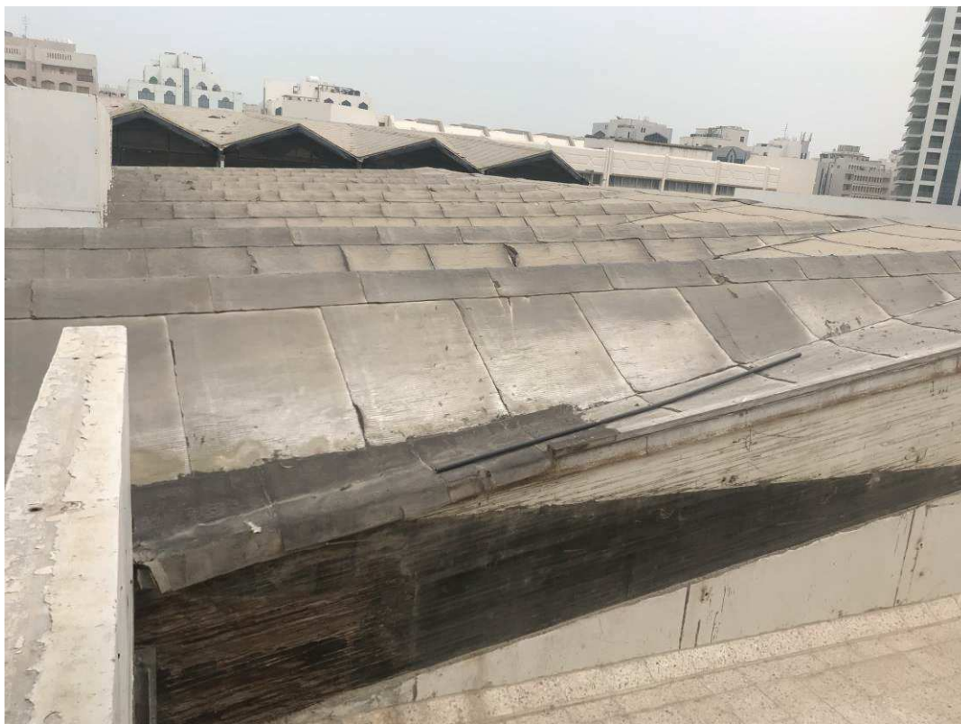
Figure 4-28 Wet rot damage in Wooden beam
