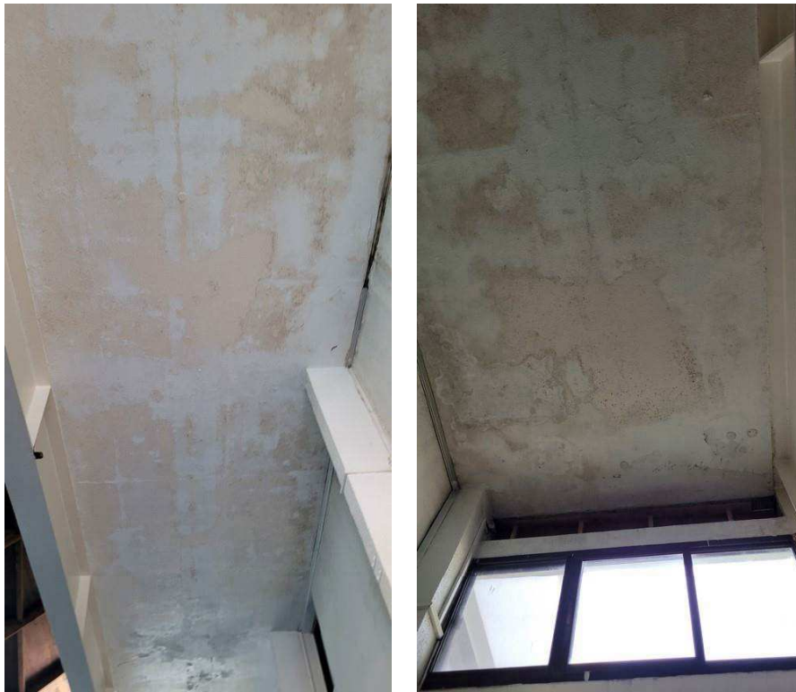
Figure 4-89 Previous leakage in slab soffit
