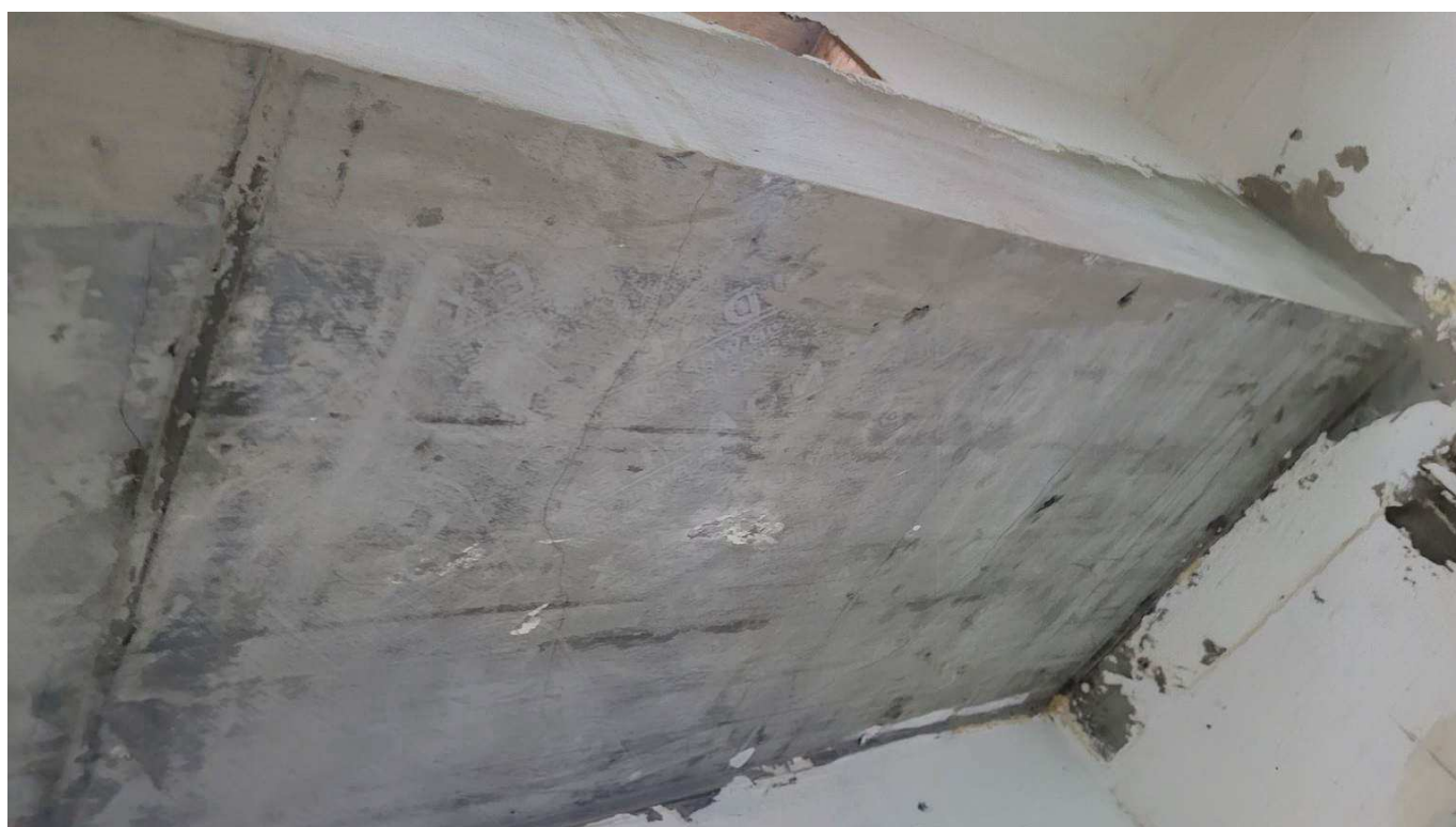
Figure 4-56 Cracks in stands soffit
