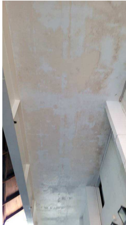
Figure 4-87 Previous leakage in slab soffit
