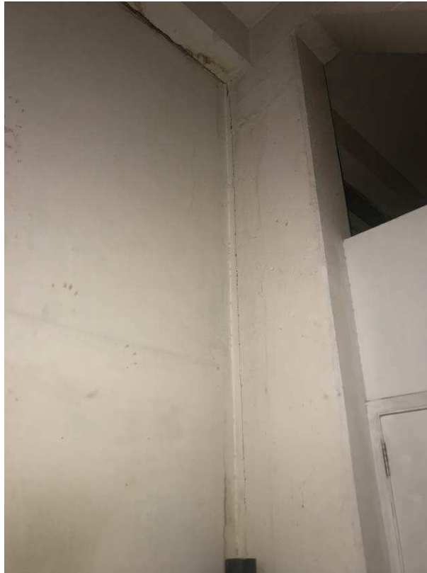
Figure 4-34 Crack between block wall and concrete element.
