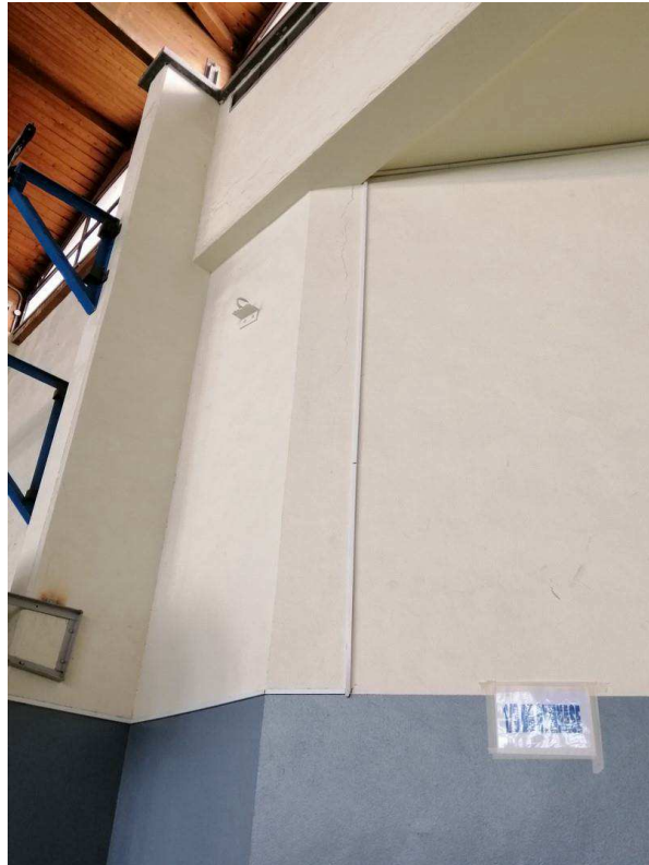
Figure 4-61 Cracks between Block wall and concrete element
