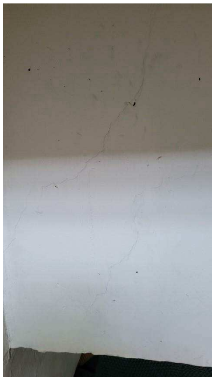
Figure 4-69 Cracks in stands soffit
