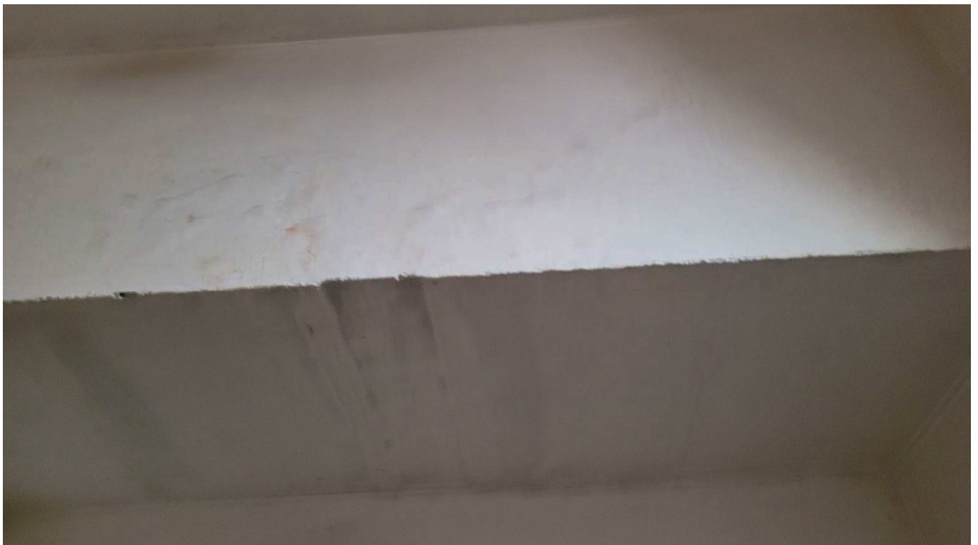
Figure 4-68 Previous leakage in stands soffit
