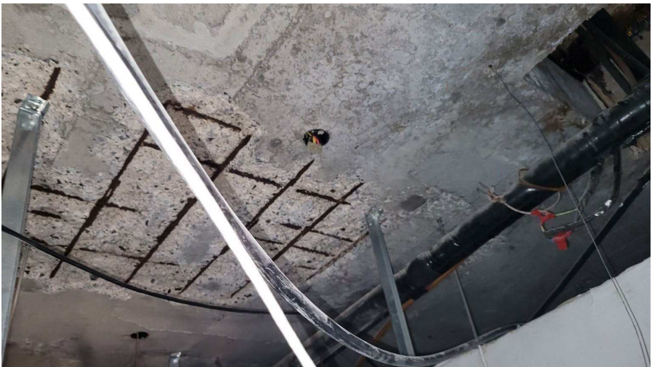
Figure 4-10 Steel exposure with corrosion in slab soffit
