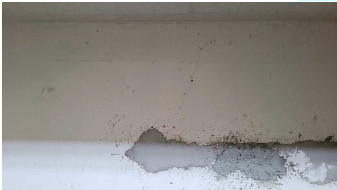
Figure 4-71 Cracks in stands soffit
